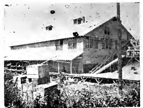
A three-story packing and storage house. The packing room containing the windows is entirely separate from the storage, a very desirable feature. The air intakes are located under the loading platform. Note the two large outlet flues.
