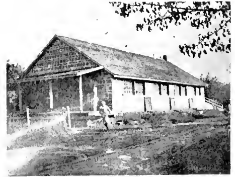
Packing room above, with storage below. The air intakes to the basement (where the shutters are lifted) are sufficiently large. The small outlet flues in the crown of the roof are entirely inadequate.
