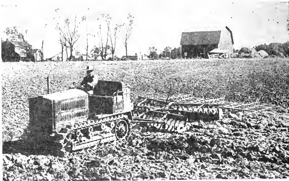
A Five-Ton Holt Pulling a Double Disk and Drag Harrow.
