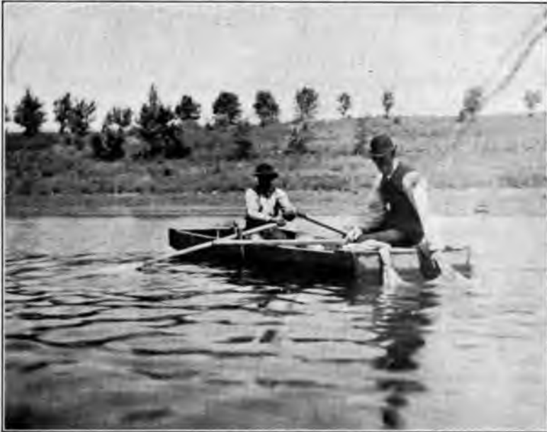
FIG. 3.—Distribution of copper sulphate. (Courtesy of W. A. Taylor, Bureau of Plant Industry, U. S. Department of Agriculture.)
