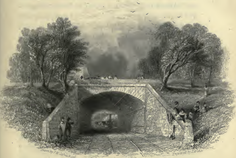
ARCH UNDER MILITARY ROAD NEAR NAWORTH CASTLE
