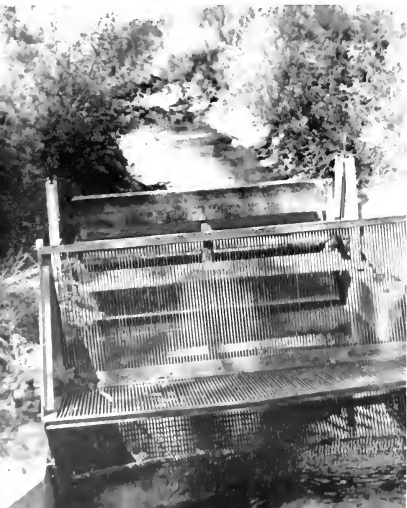
Oregon type fish screen with rotating grills—self-cleaning.
