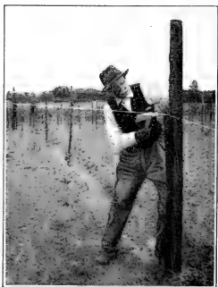
STAPLING A STRETCHED WIRE IN PLACE
