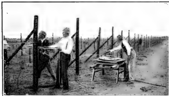
STRINGING WIRE, AND STRETCHING IT WITH A BLOCK AND TACKLE
