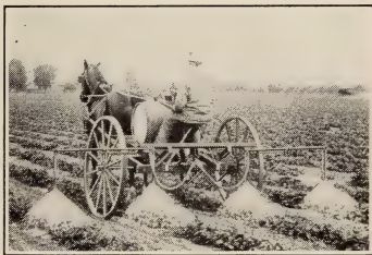
A FOUR-ROW COMPRESSED-AIR MACHINE FOR LARGE AREAS
