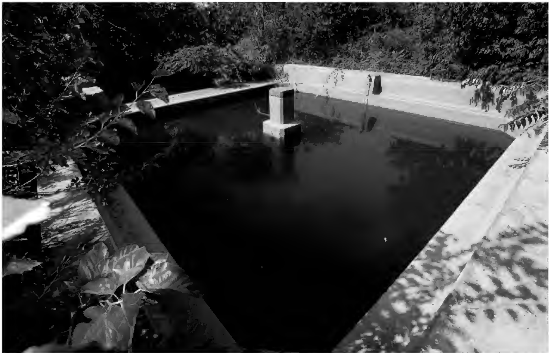
Figure 17. "Ru gebbi" (two gebbie) at Fondo Santacolomba formed by two intercommunicating water tanks.
