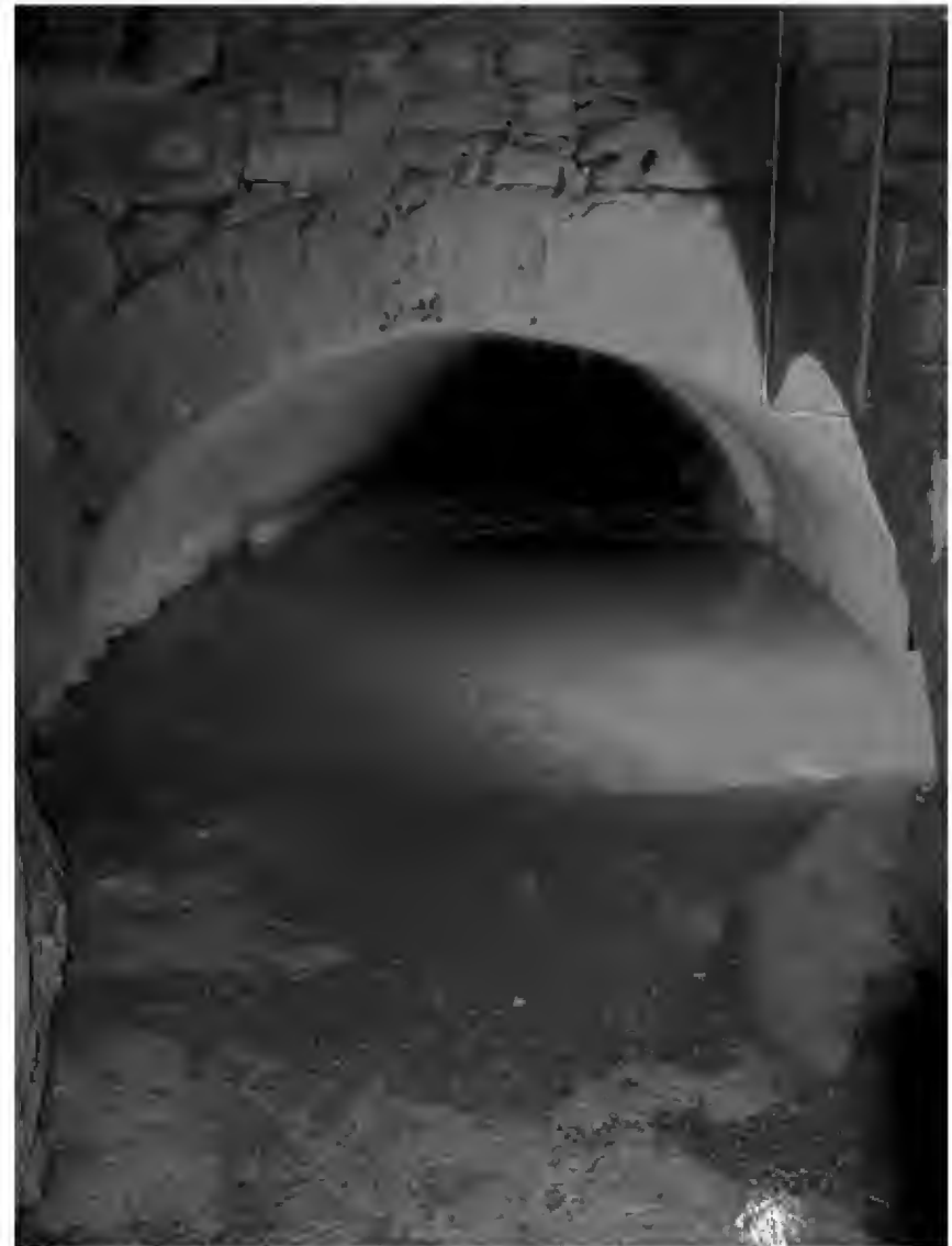
Figure 10. Detail of the Gabriele springs, now covered by an ancient structure.
