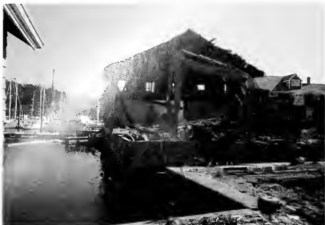
The demolition of the Carpenters' Shop.
