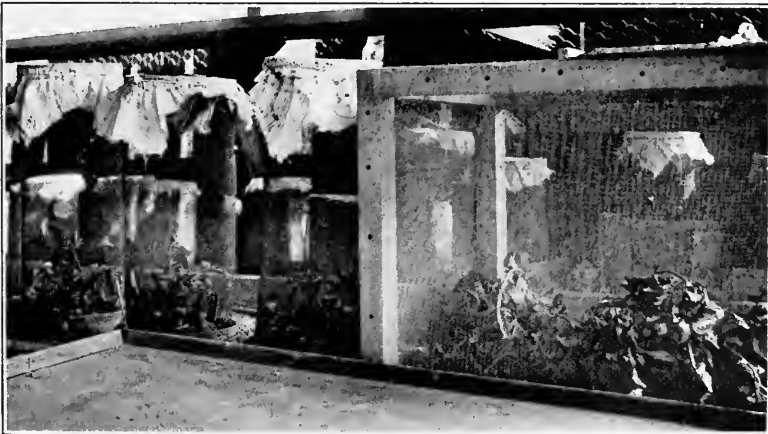
FIG. 1. Types of cages used in the food experiments. This figure shows two types: (1) circular cages composed of flower pots sunk in the soil with mosquito wire tops; (2) large oblong cages constructed of inch pine, covered with mosquito wire and set on the surface of the soil. Foliage was kept fresh in the cages by inserting them in vials of water.
