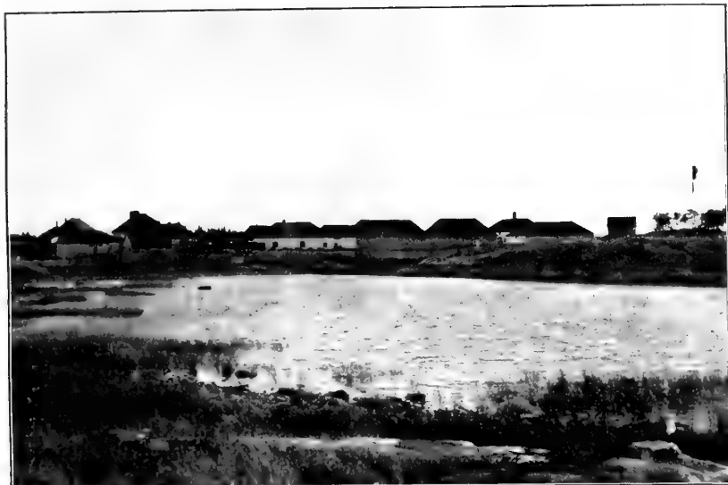
FIG. 1.—GENERAL VIEW OF NORWAY HOUSE.
