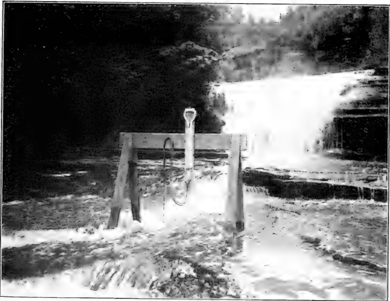
Fig. 2.—Pitot-tube as used in Cascadilla Creek
