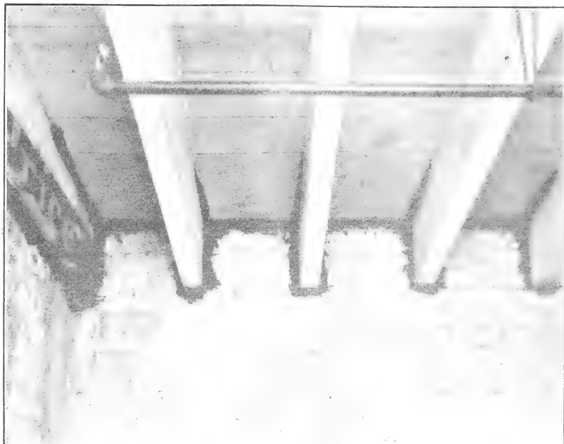
FIGURE 16.—Eaves of a tobacco warehouse sealed with plastic cement from the inside of the building. This cement was forced with a pressure gun into any crevices through which the fumigating gas might escape.
