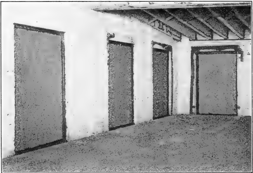
FIGURE 18.—A gasproof tar paper used for sealing the entire window space in a tobacco warehouse.
