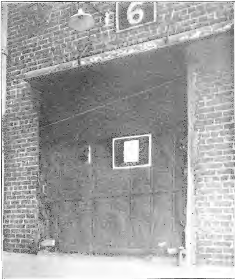
FIGURE 19.—Sliding door of a tobacco warehouse sealed with a mixture of asbestos and calcium chloride in preparation for fumigation.
