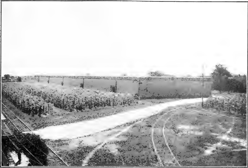
FIGURE 13.—Closed tobacco-storage warehouse one story high, divided into sections by fire walls. This warehouse was fumigated periodically during 1932 for the control of the tobacco moth.
