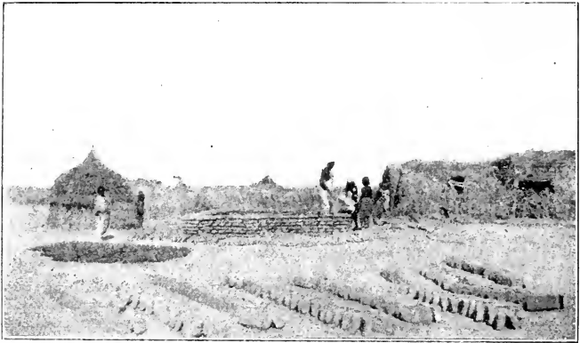
BUILDING A SQUARE BRICK HUT.
