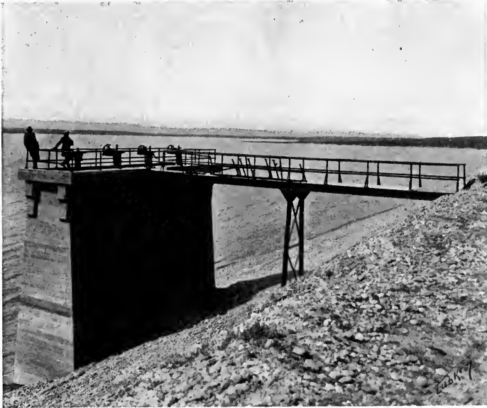
Outlet Gates at Deer Flat Reservoir, Boise Reclamation Project
