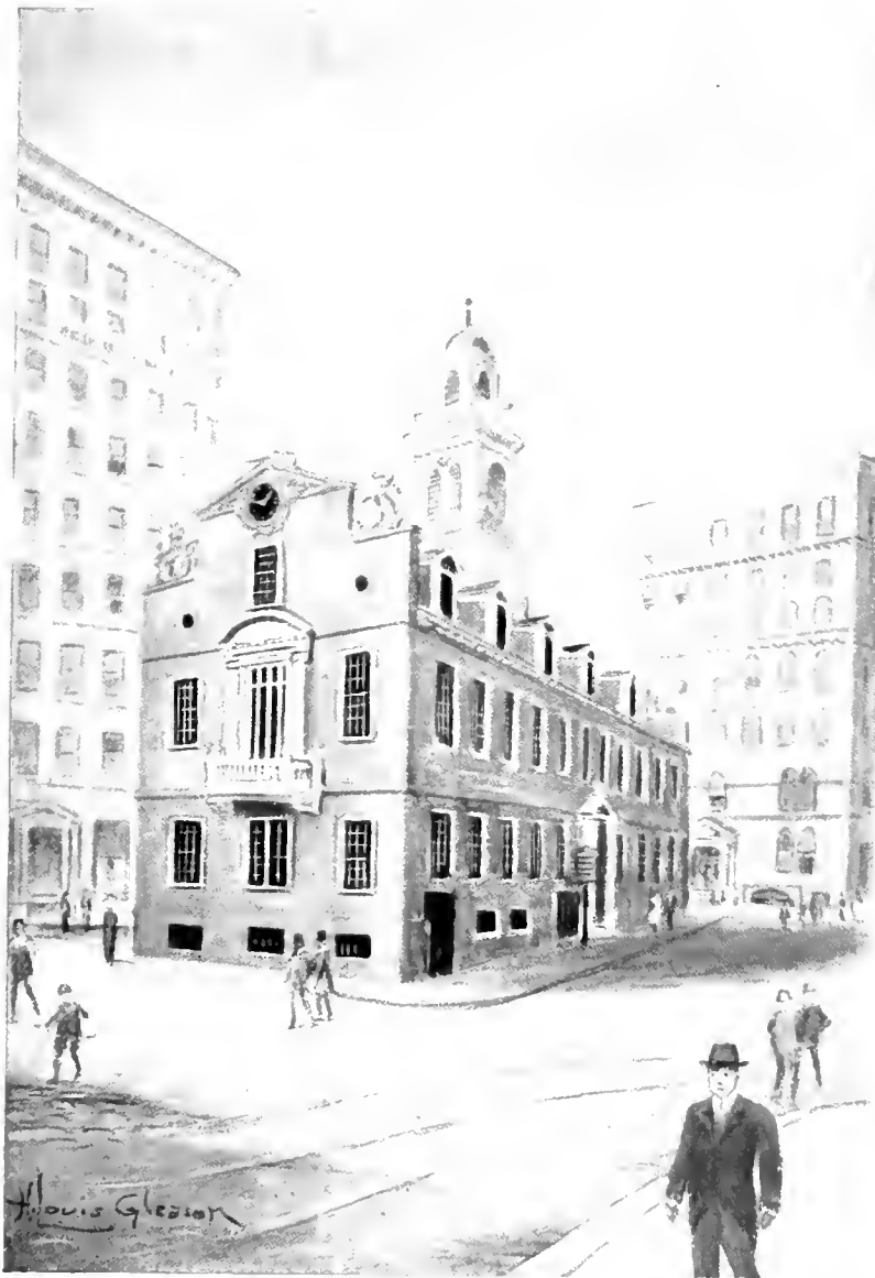
THE OLD STATE HOUSE AS IT APPEARS TODAY AMID ITS MODERN SURROUNDINGS
