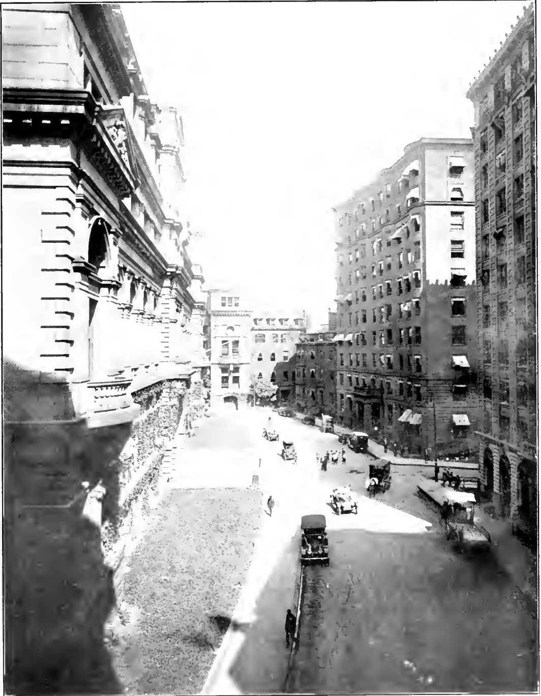
PIMBERTON SQUARE, LOOKING NORTH, THE COURT HOUSE ON THE LEFT AND OFFICE BUILDINGS ON THE RIGHT, LARGELY TENANTED BY LAWYERS AND COURT OFFICIALS
