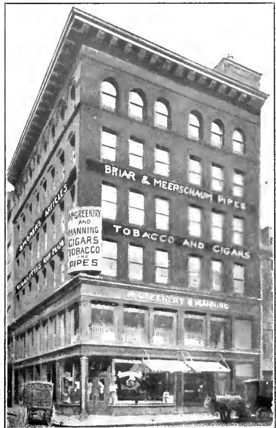
FORMER LOCATION OF THE JOSEPH P. MANNING CO., 24 FULTON STREET
