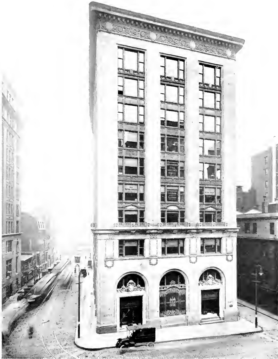
MERCHANTS NATIONAL BANK BUILDING, 28 STATE STREET
