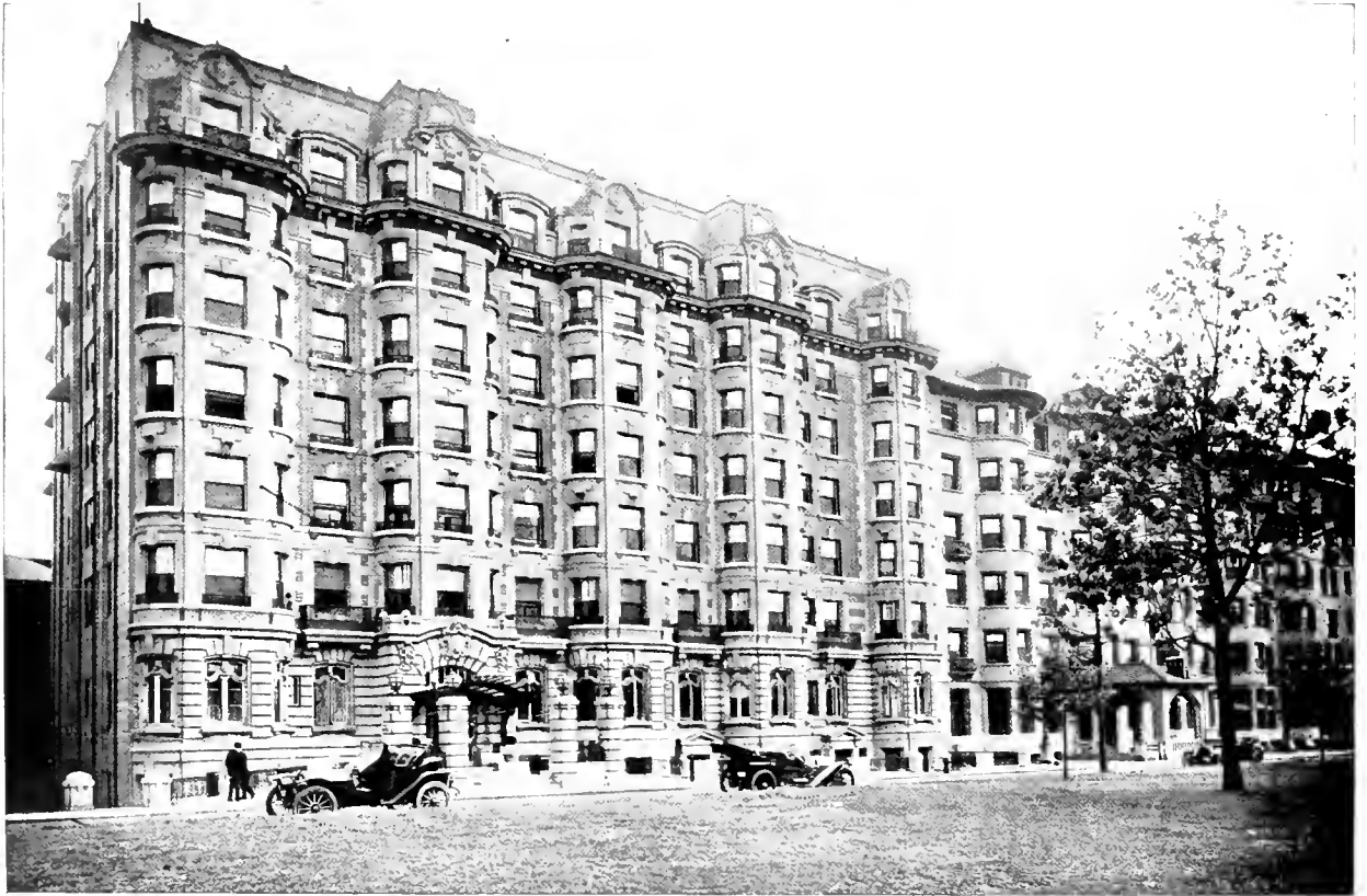
HOTEL PURITAN, 390 COMMONWEALTH AVENUE
