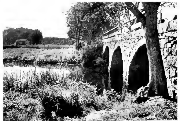
PAUL'S BRIDGE AT MILTON
