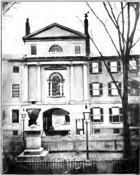
FRANKLIN STREET OF 1855, SHOWING THE SITE OF THE BOSTON LIBRARY OF THOSE DAYS. THE ARCHWAY IS WELL REMEMBERED BY BOSTONIANS OF TODAY
