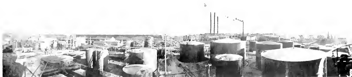
INDIAN REFINING COMPANY, GEORGETOWN, KENTUCKY, WHICH WAS RECENTLY DISMANTLED BY THE SWIFT-McNUTT CO.
