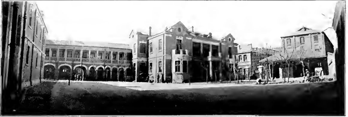
OFFICES AND GO-DOWNS OF THE CHINA-AMERICAN TRADING CO., TIENSIN, CHINA
