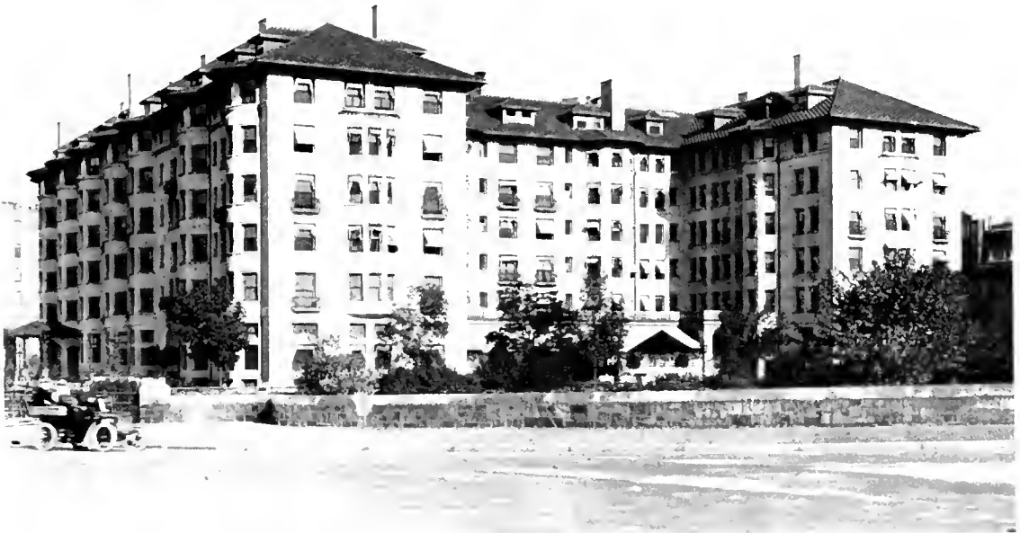
HOTEL SOMERSET, COMMONWEALTH AVENUE
