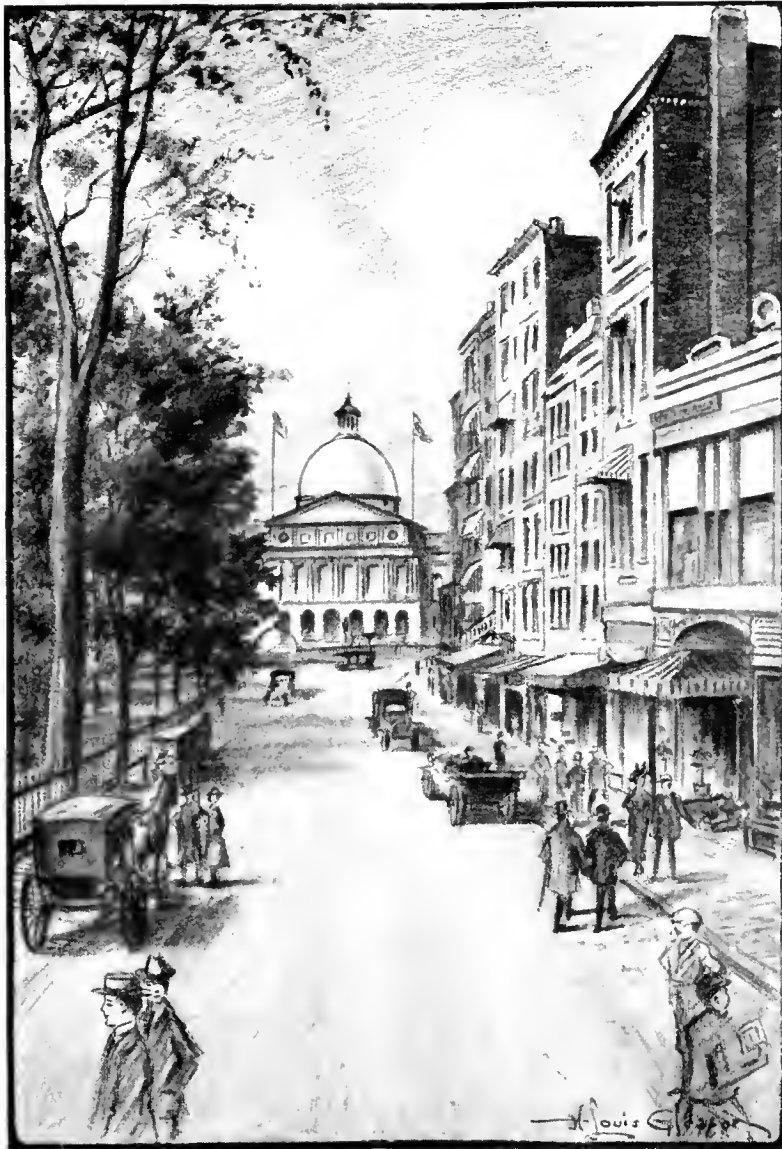
PRESENT DAY VIEW OF PARK STREET AND THE CAPITOL THE COMMON ON THE LEFT. THE BUILDINGS ON THE RIGHT NOW GIVEN OVER TO BUSINESS HAVE BEEN PROMINENT IN THE CITY'S HISTORY
