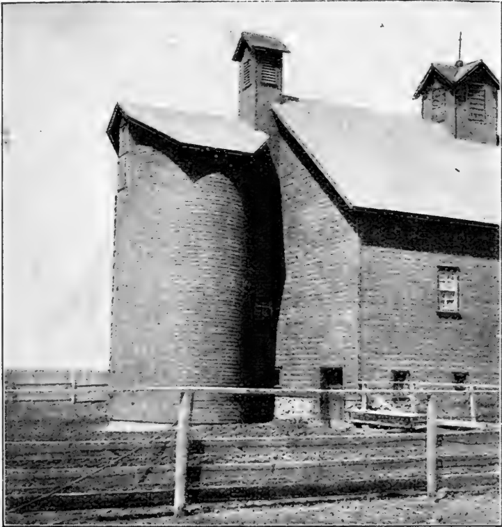
FIG. 20. ROUND WOODEN SILO, SOUTH DAKOTA AGRICULTURAL EXPERIMENT STATION.
