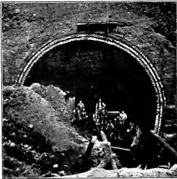
HOOSAC TUNNEL UNDER CONSTRUCTION, 1871
