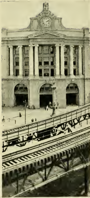
ENTRANCE TO SOUTH TERMINAL STATION.
