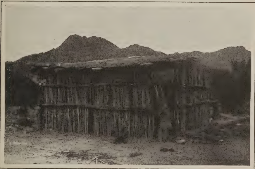
Papago house built of ribs of saguaro ( Cereus giganteus ) with corner-posts of mesquite ( Prosopis ), near Desert Laboratory.
