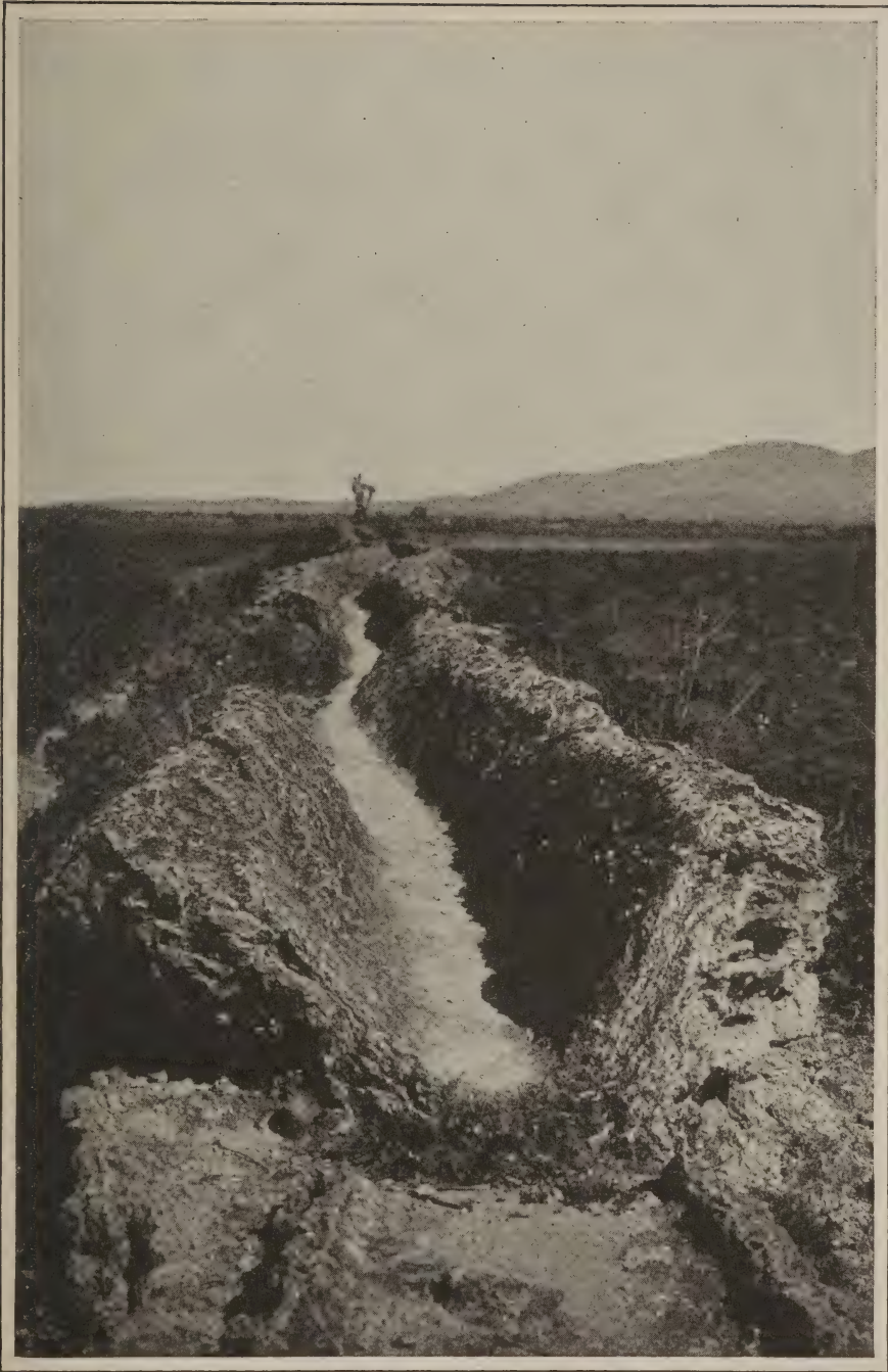
Abandoned irrigating ditch near El Riego, Tehuacan. The walls have been built up by lime deposits until the conduit became useless, and it has been cut for a roadway.
