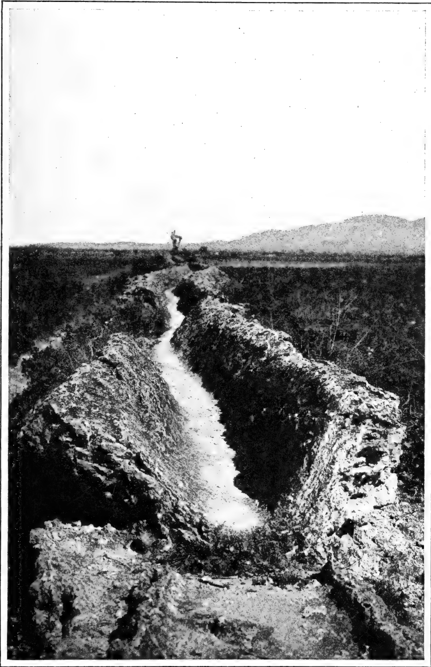
Abandoned irrigating ditch near El Riego, Tehuacan. The walls have been built up by lime deposits until the conduit became useless, and it has been cut for a roadway.
