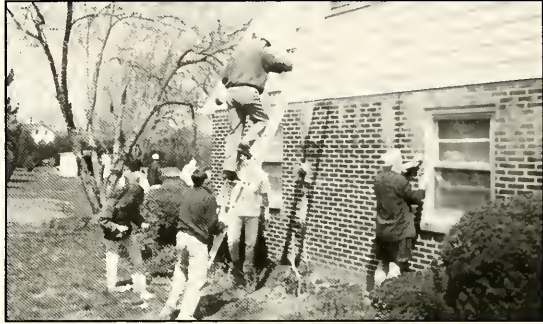
Project crew busy scraping, sanding and painting
