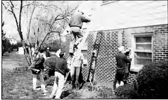
Project crew busy scraping, sanding and painting
