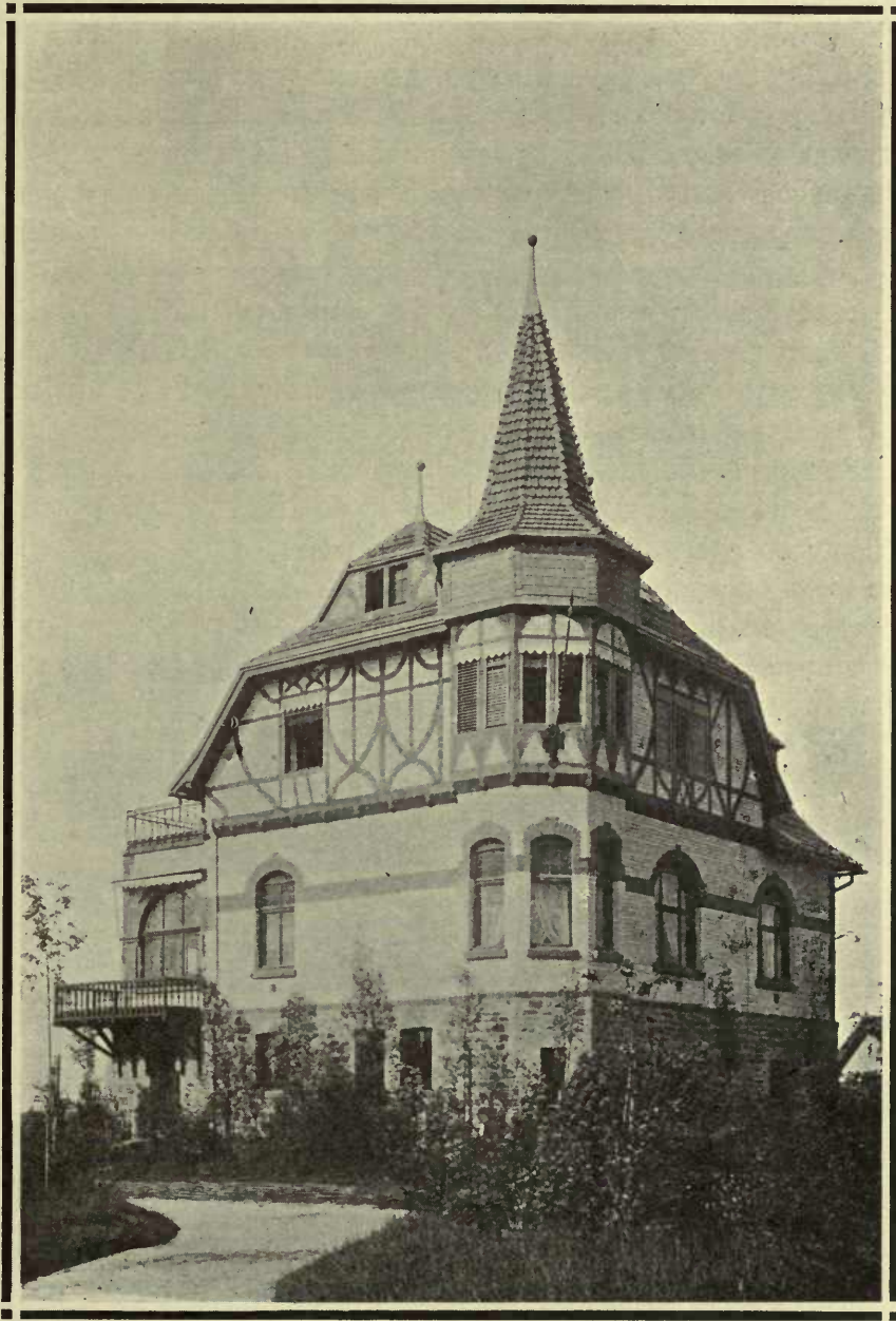
FIG. 62. Villa Built of Lime-Sand Bricks
