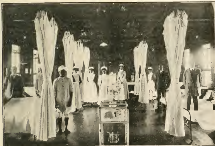
A Ward in the Native Hospital. Grey's Hospital, Pietermaritzburg.
