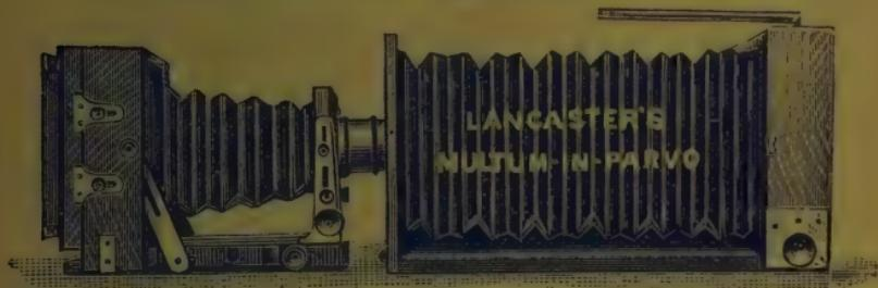
**FOR ENLARGING.**—The Negative must be placed in a Dark Slide of ordinary Camera, and the enlargement taken in Multum-in-Parvo, the plate going into the end of Camera.
