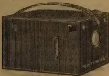
for examination, and we find that by moving a lever it acts automatically without a hitch. It takes plates as well as films—a fewer number of the former, of course. The movement of the one lever releases the exposed film, and sets the next one ready for exposure. The mechanism is exceedingly simple and not likely to get out of order. We predict great popularity for the new camera.
