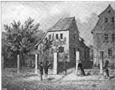
Schillerhaus in Gohlsis
