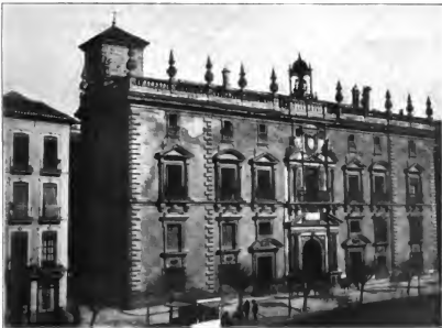
Abb. 43 Chancilleria in Granada Fassade
