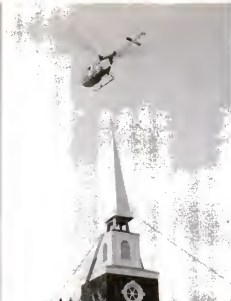
3. STILL FLYING BLIND , pilot successfully drops steeple in place on his fourth attempt.
