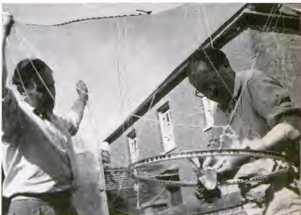
CAMERA SUPPORT is a bike wheel with spokes removed and rim drilled to keep weight to minimum. Most photos are shot with wide-angle 80-deg. lens at f/16 , 1/500 sec., medium-fast film.
