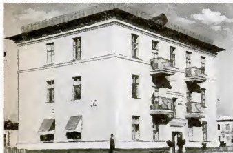
ANTI-SEISMIC HOUSE is said to be able to resist 36-hour shock. Most quakes last seconds.
