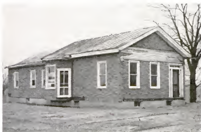
5. NOW A BUNGALOW , with second-floor waste trimmed off, house rests on new foundation.
