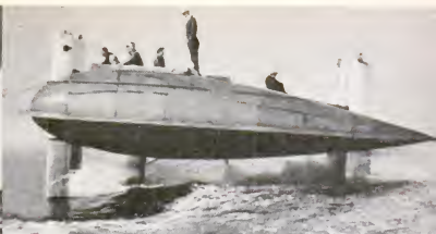
TEARDROP-SHAPED Lantern, Dr. Vannevar Bush's submerged-foil craft of early Fifties, showed stability as passenger rode erect standing. Foil-control system was ahead of its time.
