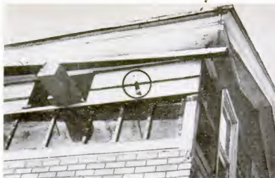
1. SAW POKES NOSE THROUGH, near one corner (circle). Its wielder is inside second story.
