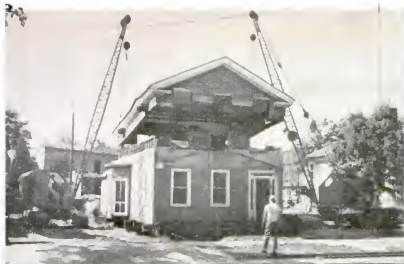
2. TWIN CRANES lift off roof. Chains secured to beams passed through wall holes held it.
