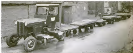
Its truck wheels down, the trackmobile hauls yard dummies.
