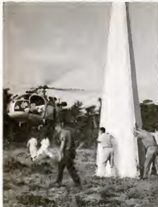
1. COPTER HOVERS 10 feet off ground while crew attaches ropes from 32-foot steeple.
