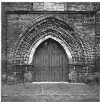
Thurm-Portal in der Westwand.
