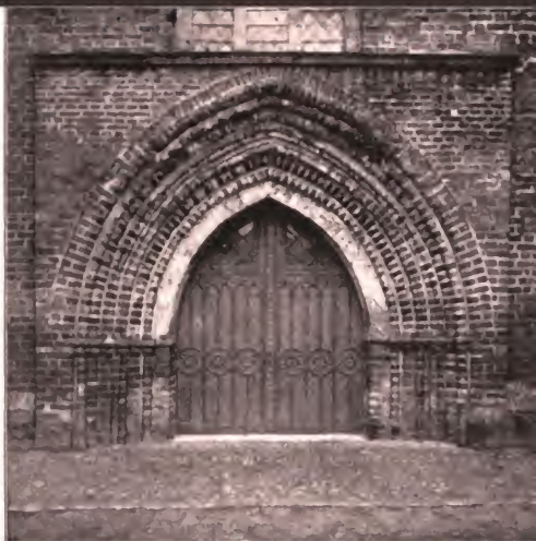
Thurm-Portal in der Westwand.
