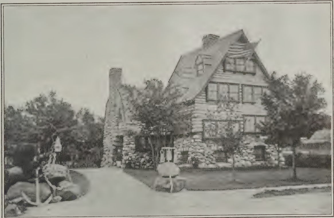
Dwelling House Originally Erected at Bar Harbor, Maine, Taken Down Stone by Stone, Transported to Kentucky and Rebuilt on Sherley Crest Farm Near Lexington
