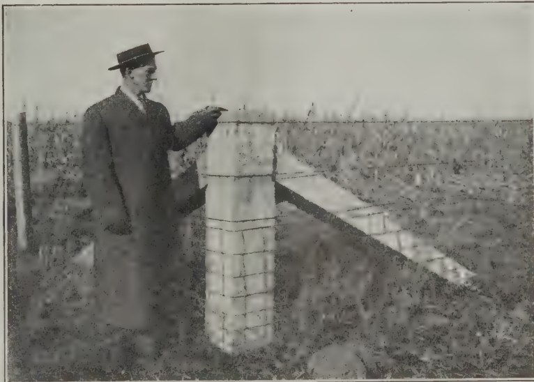
Fig. 1—Appearance of the Finished Post in Position
