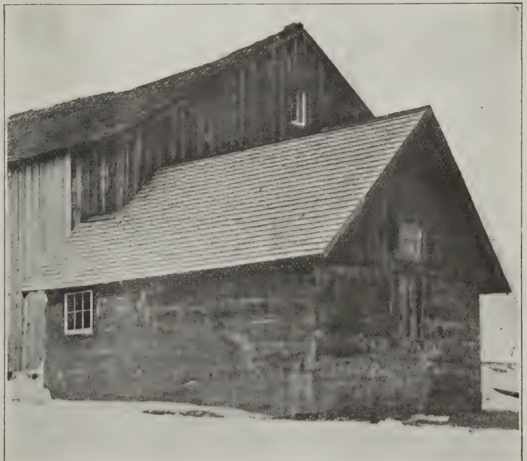
Fig. 2—Appearance of the Finished Ice House with Milk Room in the Rear
