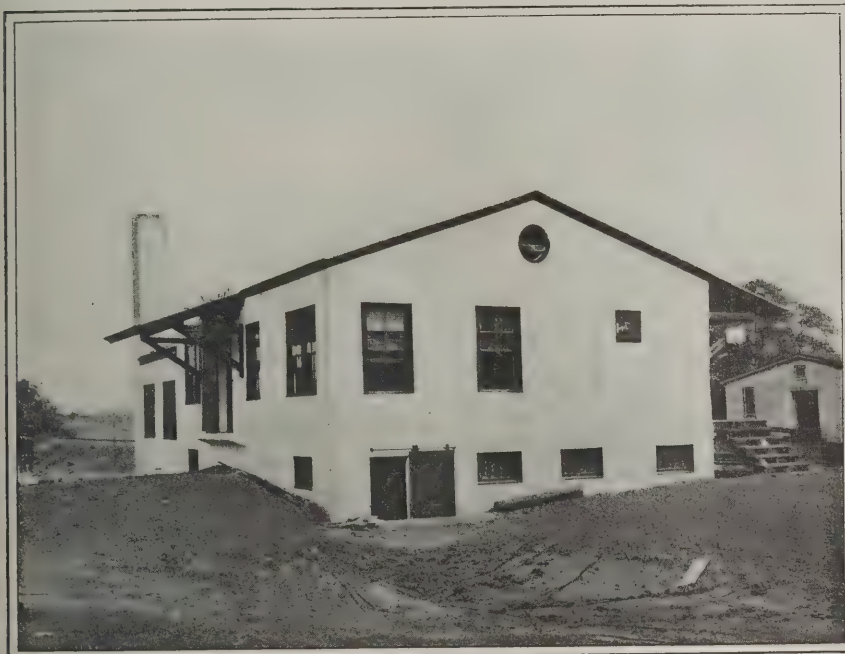
Photographic View Showing Receiving Door at the Left and Cold Room Entrance at the Front
