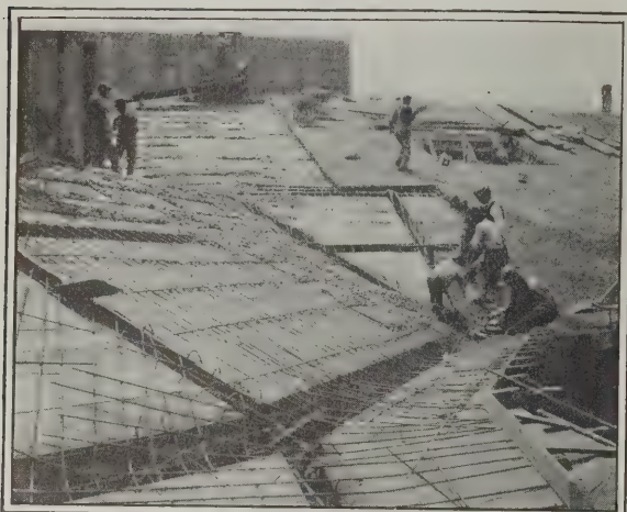
Reinforced Concrete Construction—"Pouring" a Theatre Balcony
