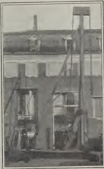
An Extemporized Building Hoist
