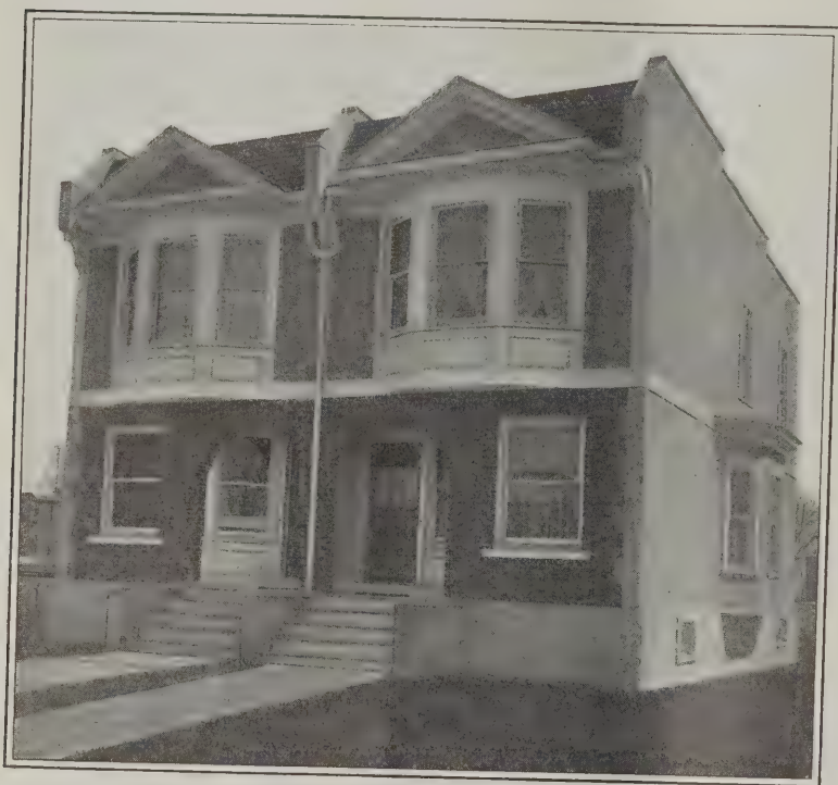
A Front and Side View of the Completed House
