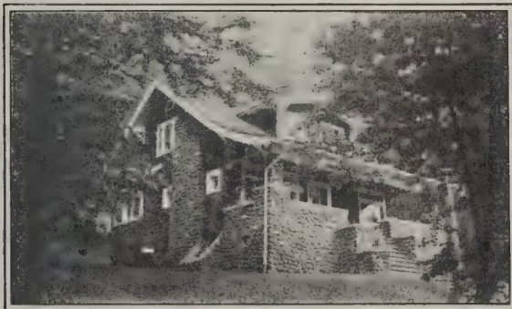
View of Bungalow Showing Cobble Stone Porch and Chimney
