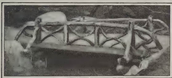
Fig. 9.—Rustic Bridge Constructed of Locust Tree
