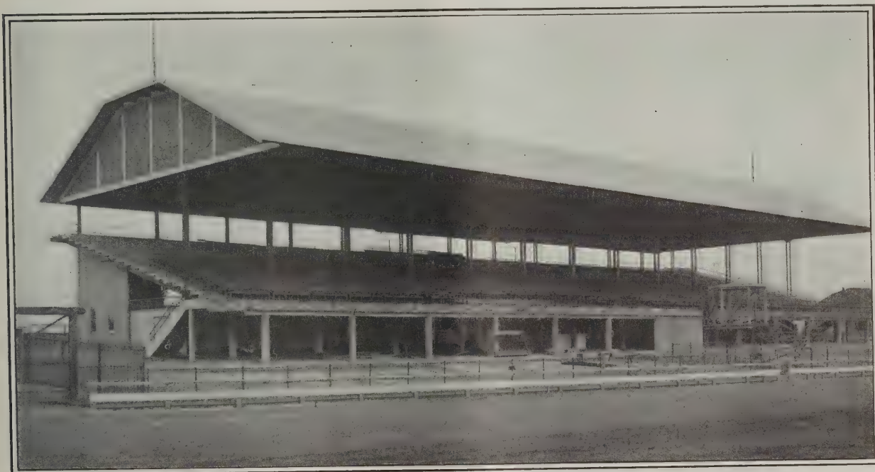
Reinforced Concrete Grand Stand of the Forest City Live Stock and Fair Co. at Randall, Ohio
