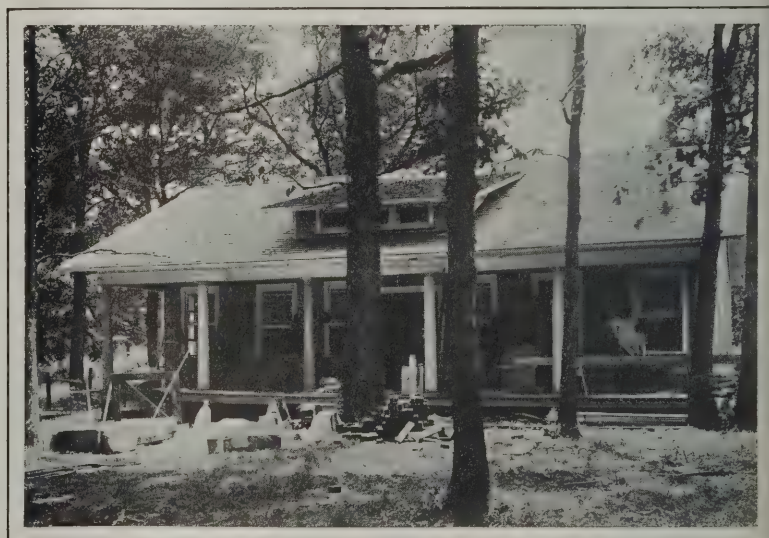
Appearance of the Camp Building When Practically Completed
