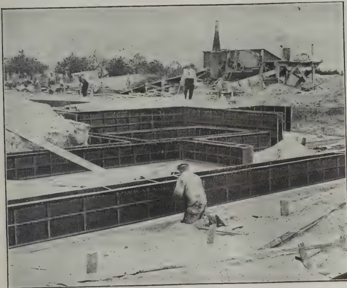
Fig. 7—The Blaw System of House Molds or "Forms"
