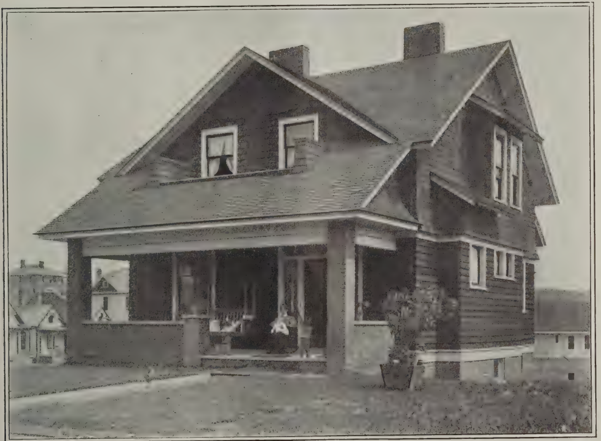
Frame Cottage Designed, Built and Occupied by P. O. Andrews, Knoxville, Tenn.
