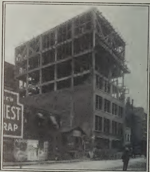
A Light Manufacturing Building in Course of Construction
