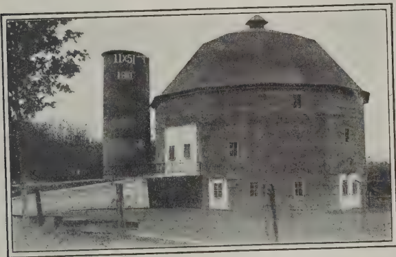
Appearance of the Barn and Completed Silo
