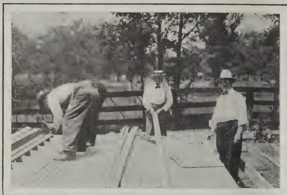
Building a Summer Camp—Members of the Builders' Exchange Laying the Floor
