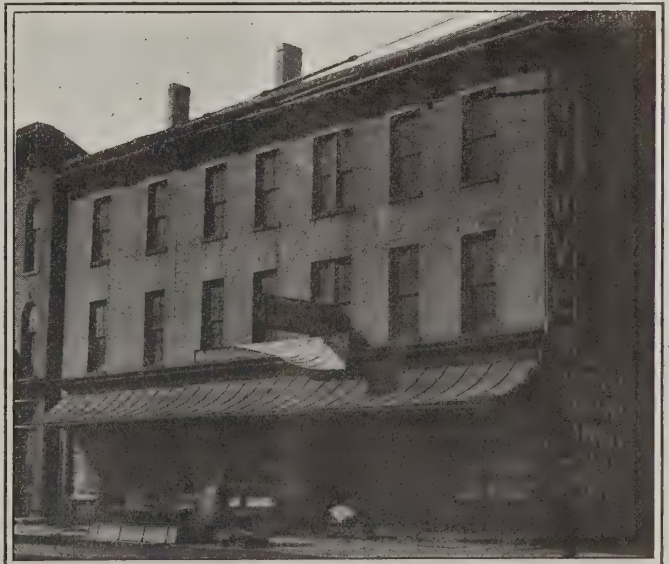
Fig. 2—The Building Before the Remodeling was Effected
