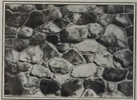
Fig. 11—An Excellent Example of "Weather" Pointing
