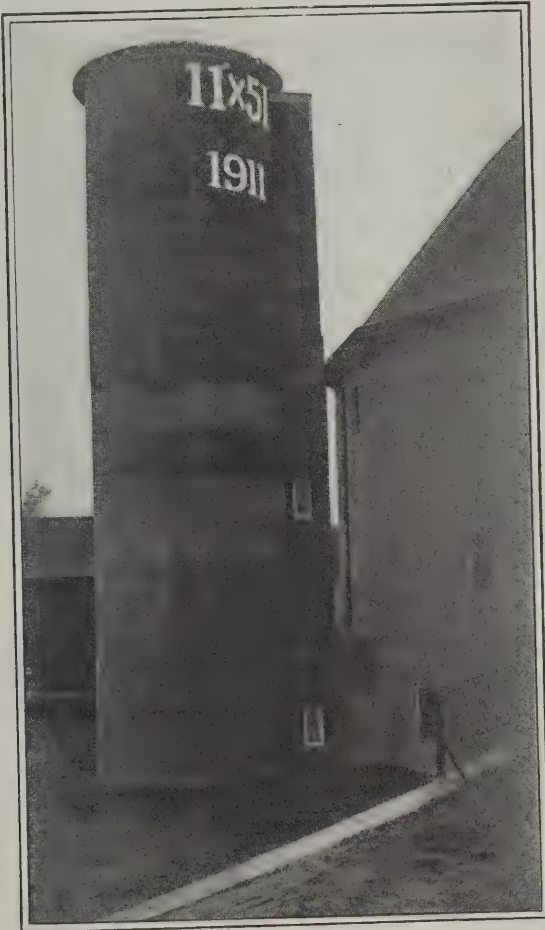
Side View of Silo, Showing Junction with the Barn
