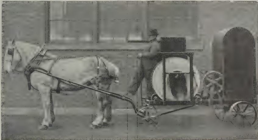
Fig. 11—The Chain Belt Concrete Mixer Showing Engine Enclosed and Horse Attached, Ready to Move to Next Job
