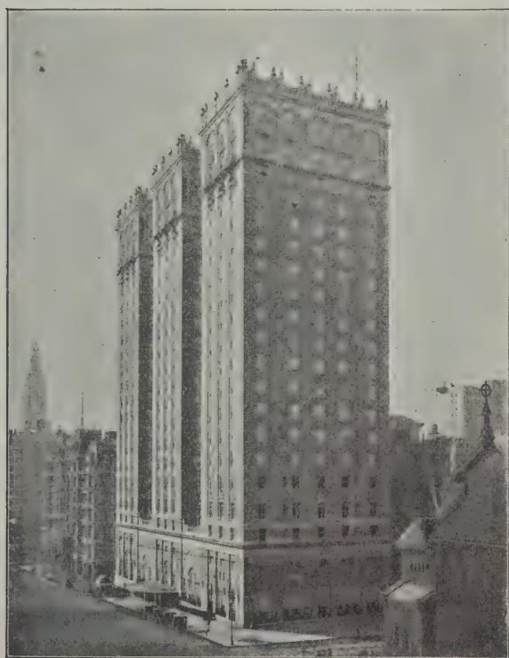
Fig. 1—General View of the New Fireproof Vanderbilt Hotel
