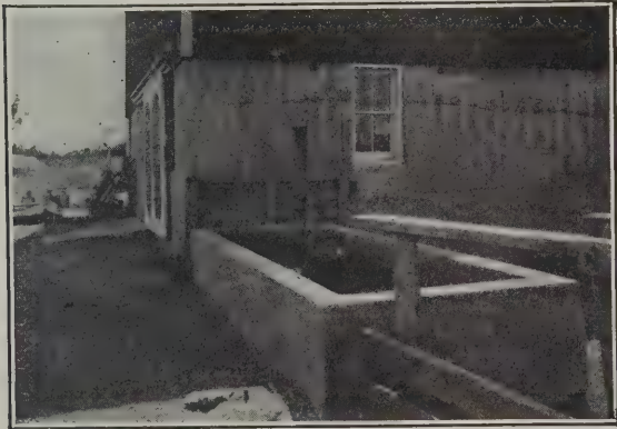
General View of the Completed Tank
