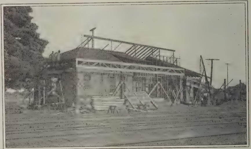
Fig. 10—Showing Some of the Details of the Remodeling
