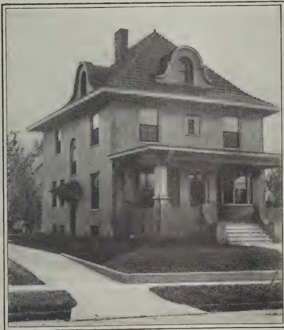
Gypsum Plaster on Metal Lath—An Interesting Example
