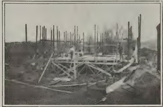
Erecting Scaffolding and Floor "Forms" Preliminary to "Pouring" the Concrete
