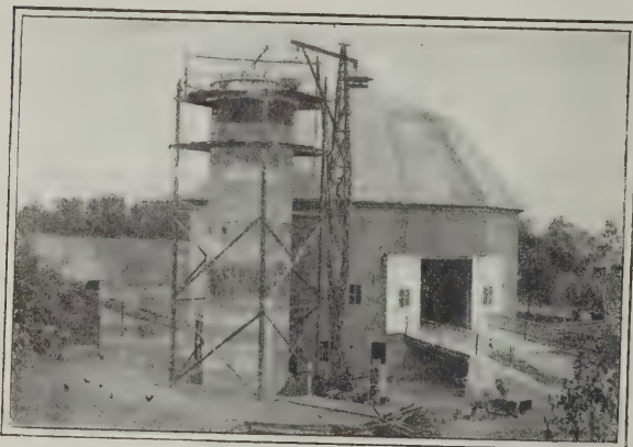
View of Silo with the Walls Completed
