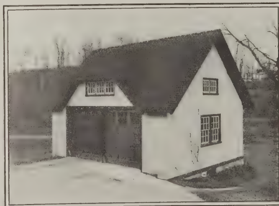
A Simple Application of Stucco
