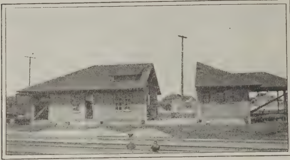
Fig. 9—Building Spread Apart and Lowered to Its Foundations
