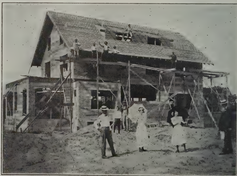
Fig. 10—Dwelling House Nearly Completed by the Van Guilder System
