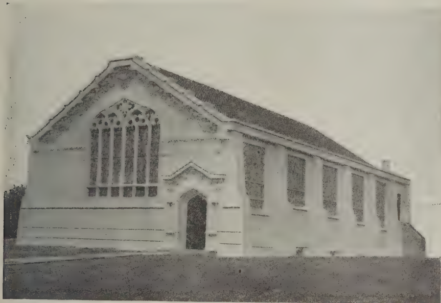
General Appearance of the Finished Building
