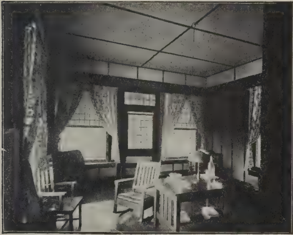
Wall Board and Its Uses—Fig. 1—Showing Application in Living Room
