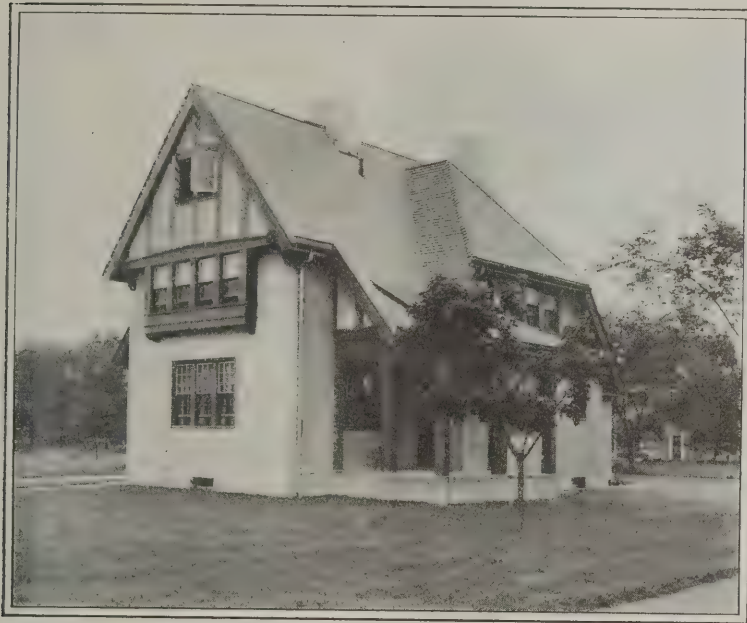
House and Garage of Stucco Exterior on Metal Lath—View of Front and Right Side of Building
