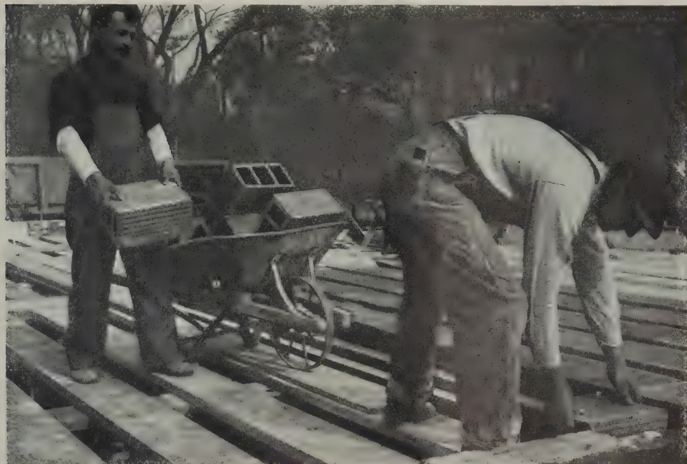
Making Men Work—Fig. 4—Seven or More Pieces of Hollow Tile are Easily Carried in a Wheelbarrow—Laying a Hollow Tile Floor
