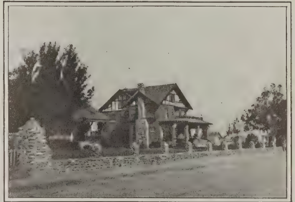
Fig. 218.—Fence Constructed of Cobblestones with Iron Chains Suspended from Pier to Pier
