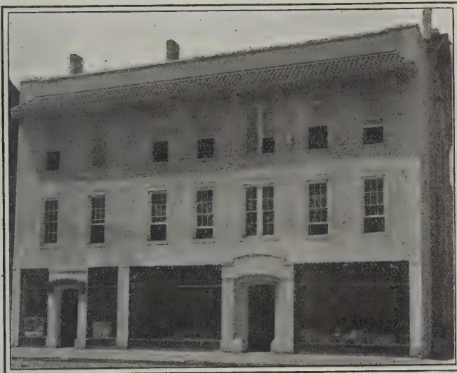
Fig. 1—Appearance of the Front of the Building After it Has Been Remodeled
