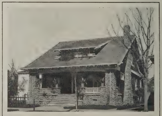
Fig. 5—A Case Where the Chimney is Built of Cobble Stones
