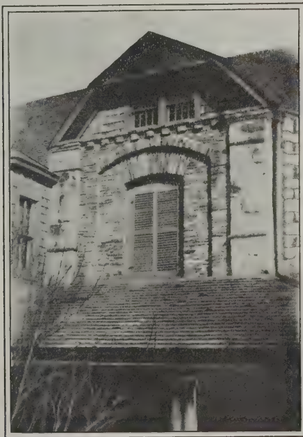
Fig. 15—A Rather Unusual Treatment Involving the Use of Common Field Stone
