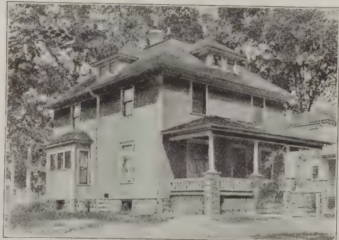
A Good Example of Stucco Construction
