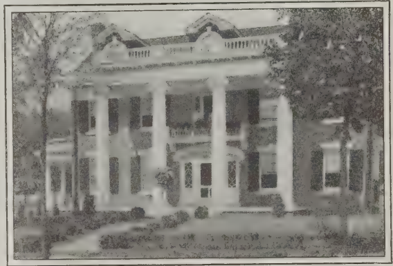
Fig. 16—Showing Use of "Koll" Built-up Columns
