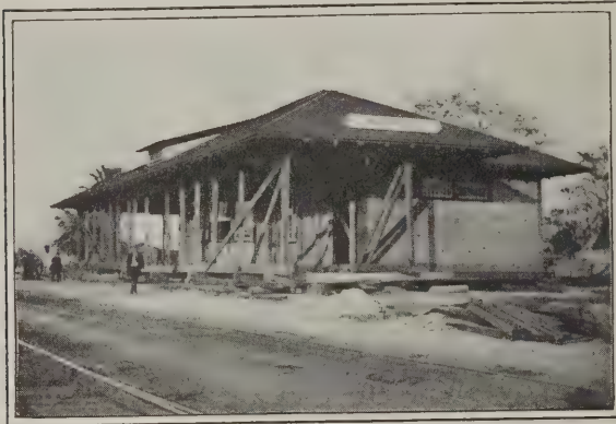
Fig. 3—View of the Building After It Had Been Moved a Little More Than its Own Length
