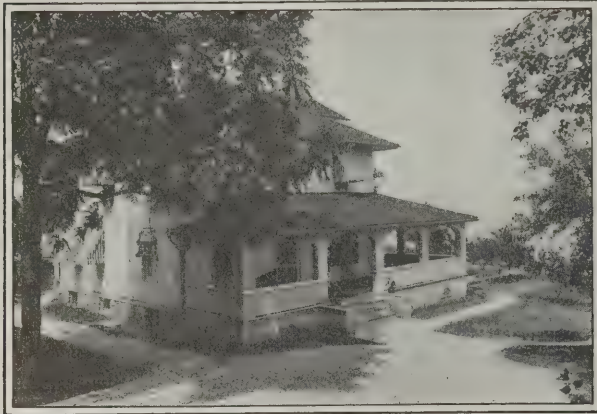
View of Rear and Side with the Hudson River in the Background
