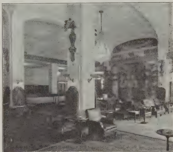
Fig. 2—Foyer in the Hotel, Showing How the Electric Lamps are Used for Decorative Lighting
