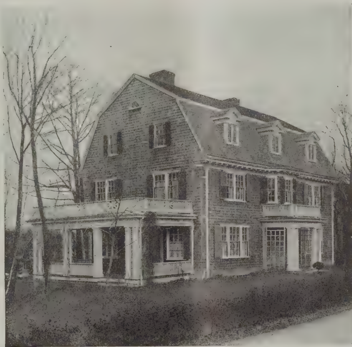
Fig. 1.—Exterior View of Residence at Newton Center, Mass., Heated by System Named
