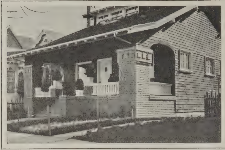
The Camera as an Adjunct of the Builder's Equipment—Fig. 9—An Excellent Example of Pressed Brick with Raked Joints
