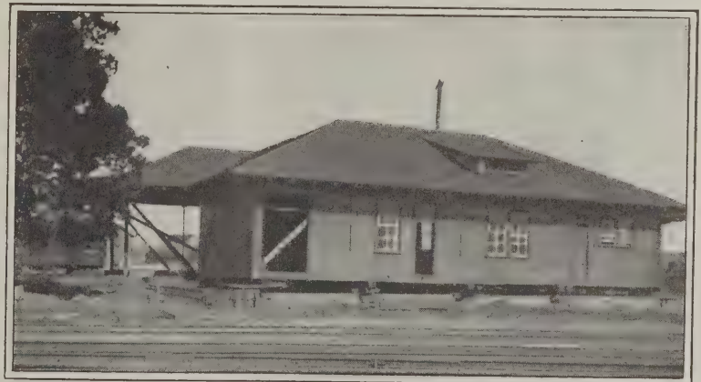
Fig. 8—Appearance of Building on Its New Foundations
