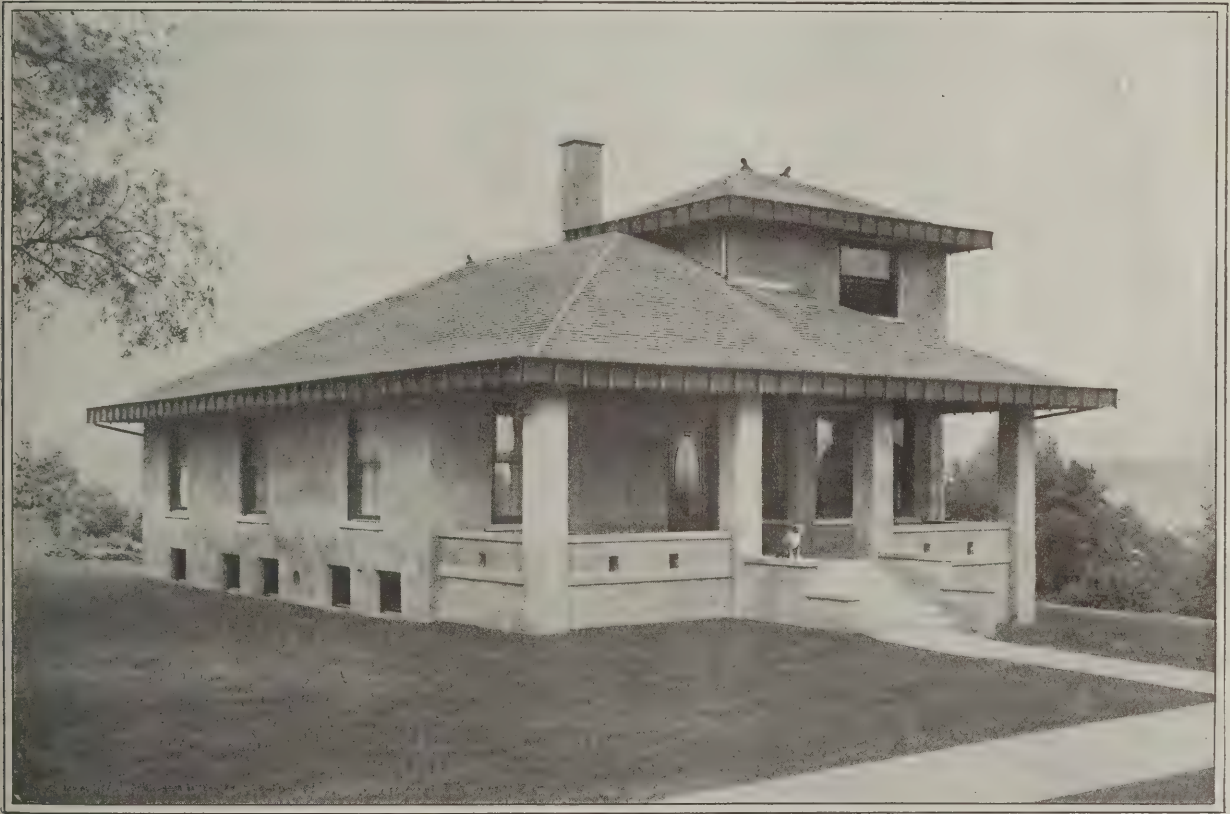
General View of the Concrete Tile House of Dr. A. A. Mahle at Lemont, Ill.
