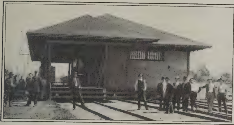
Fig. 5—Appearance of Building When Crossing the Railroad Tracks
