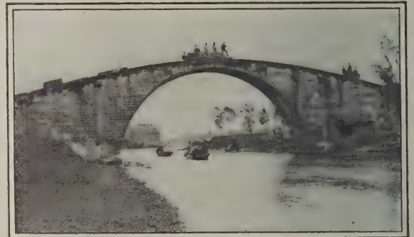
Masonry Bridge of Ancient Construction
