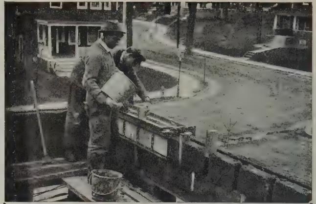
Making ready to insert the floor beams.
