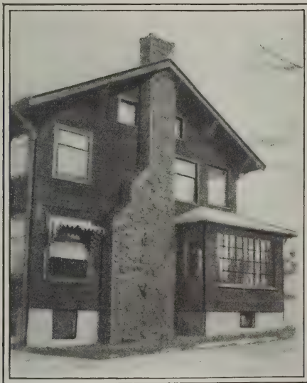
Fig. 19—A Chimney of Rough Brick
