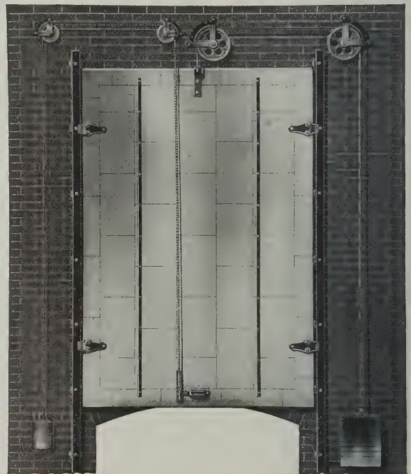
Fig. 10—Richards Vertical Fire-Door Fixture, No. 203
