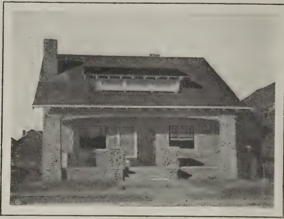
The Camera as an Adjunct of the Builder's Equipment—Fig. 3—A Good Example of the Use of Cobble Stones
