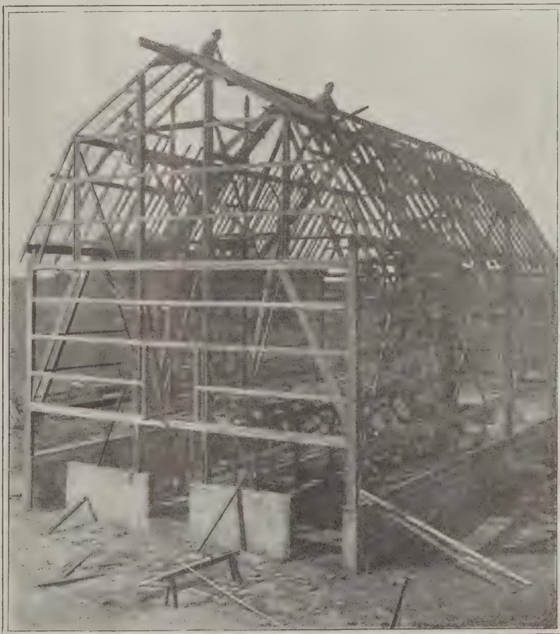
Another Barn of Plank Frame with Concrete Basement Walls
