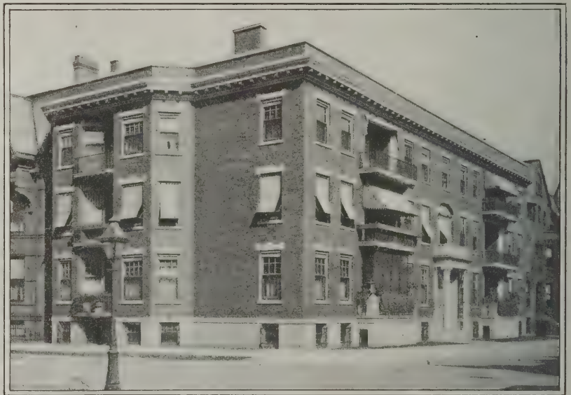
A Brick Apartment House Showing the Use of Enamelled Terra Cotta for Ornamental Purposes
