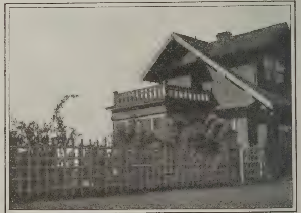
Fig. 214.—Fence Built of Rough Lumber
