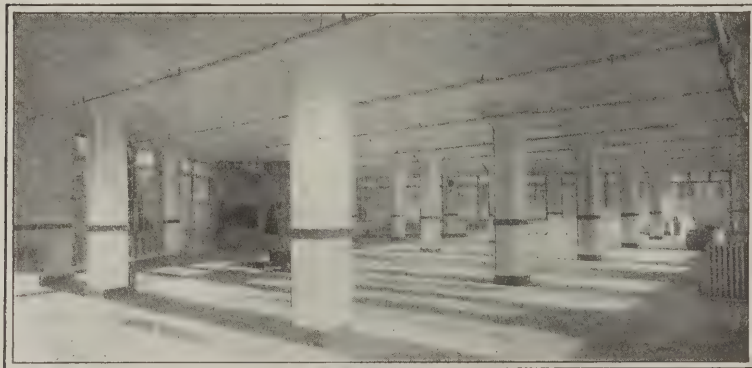
Interior view on one of the floors of the factory building
