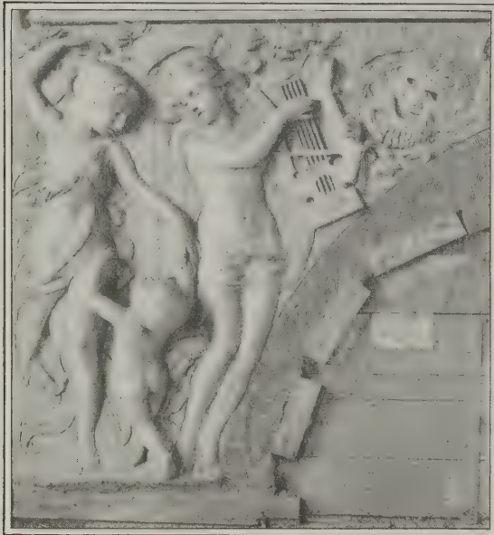
Artistic Use of Terra Cotta in Home Building—Detail of a Decorative Spandrel
