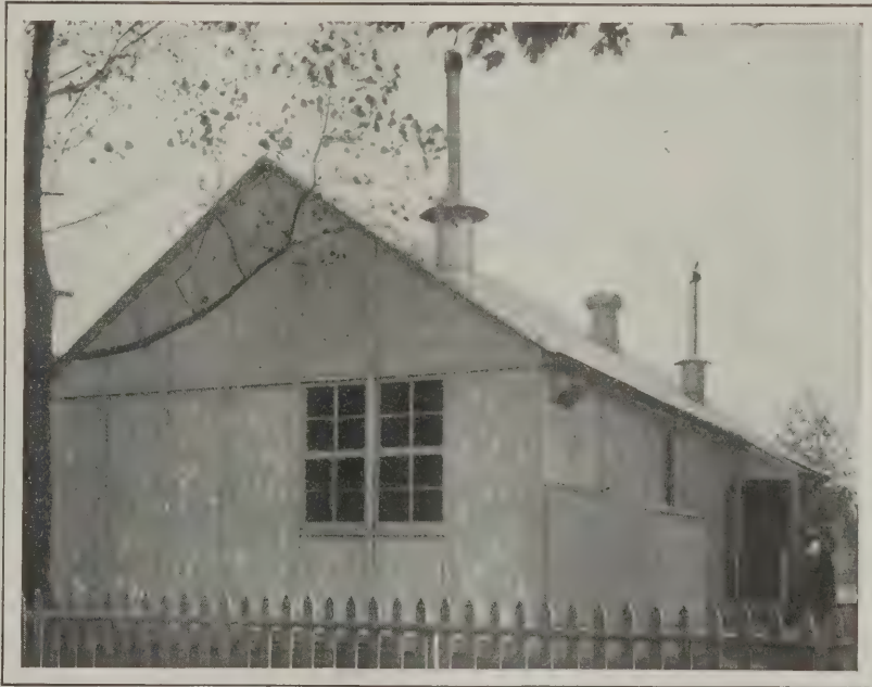
Exterior View of the Portable Building Showing Position of Chimneys and Ventilator
