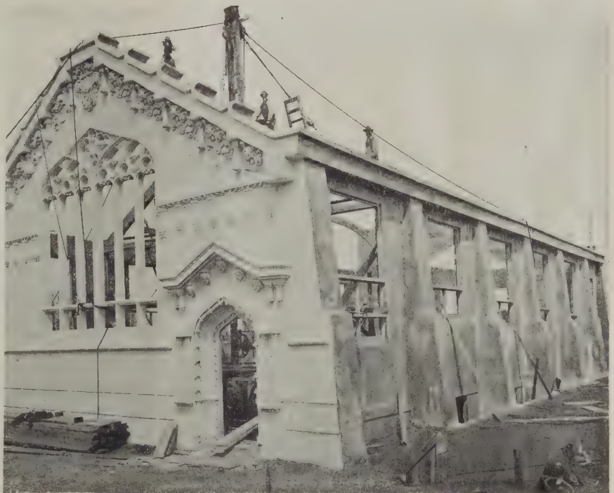
View of Building After the Four Walls Had Been Erected and the Corners "Poured"
