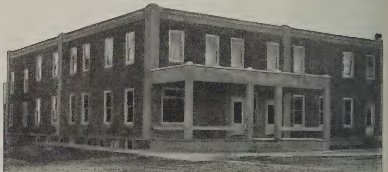
Fig. 11—Example of a Cement Over-Coated Building
