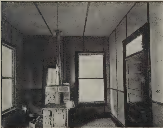
Fig. 2—Interior of Kitchen Finished with Wall Board
