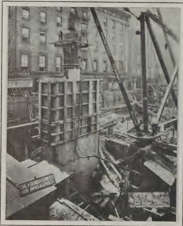
Showing a Caisson Being Sunk for a Foundation Pier.
