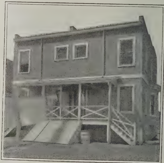
A View at the Rear of the Building
