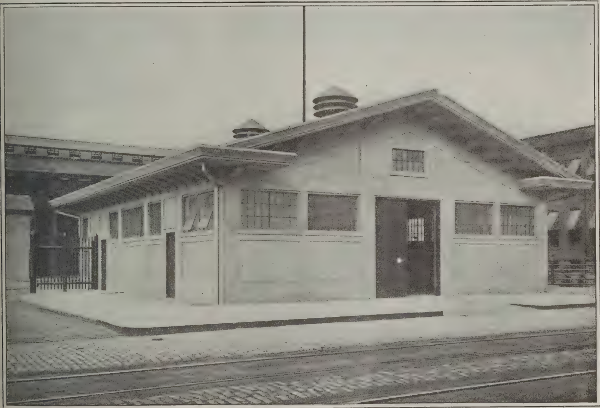
General View of the Concrete Building as Erected by the National Tube Company at McKeesport, Pa.
