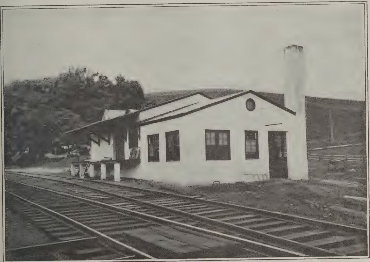
Photographic View of the Building With Boiler Room End in the Foreground
