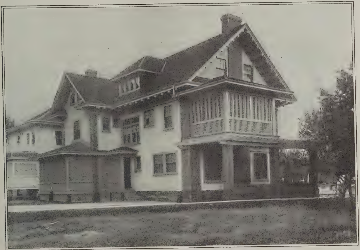
Photographic View Showing the Rear and End of the House; also the Enclosed Porch
