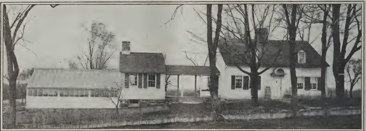
Fig. 11—Showing How an Even-Span Greenhouse Can be Attractively Arranged as an Extension to a Country Dwelling
