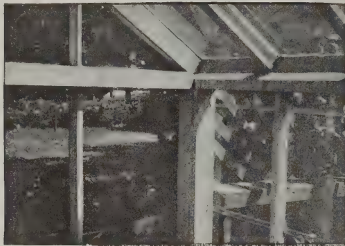
Building a Small Greenhouse—Fig. 4—Corner Framing
