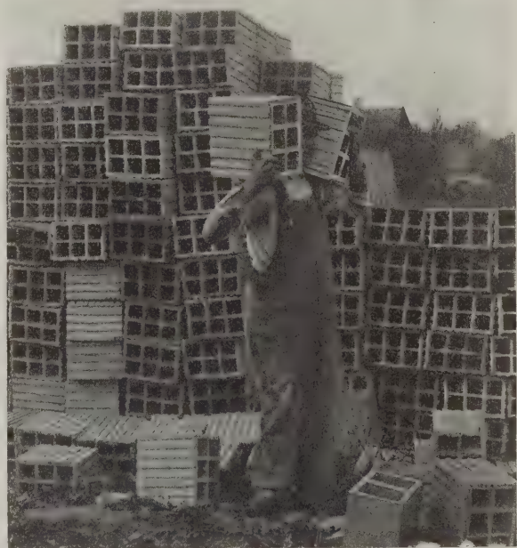
Fig. 5—Not the Right Way to Handle Hollow Tile Efficiently
