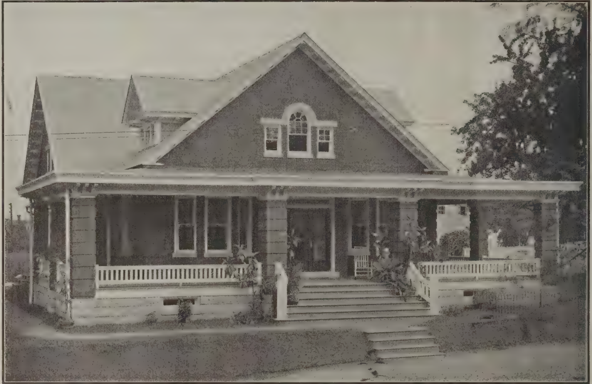
Bungalow of Unas. S. Buz, Harrisburg, Pa., Kooted with Ambler Asbestos "Century" Shingles. Architect, H. F. Conover, Washington, D. C. Contractor, John Meyers, Harrisburg, Pa.
