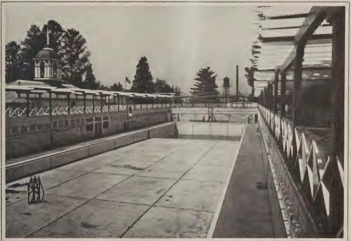
General View of Open Air Swimming Pool As It Appears Free from Water—Designed by D. X. and J. C. Murphy, Louisville, Ky.
