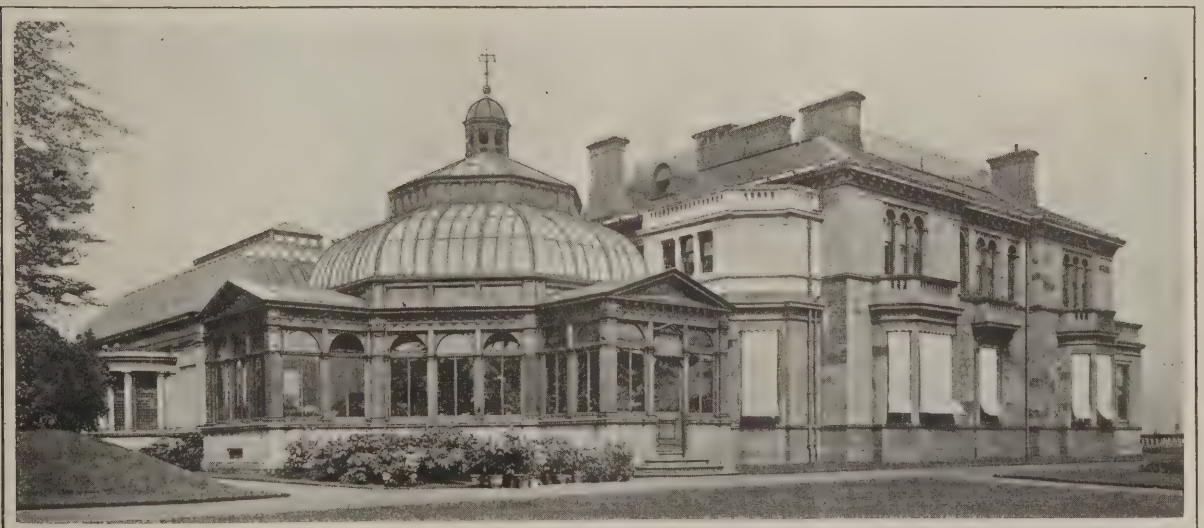
Fig. 3—Showing an Octagonal Domical Conservatory with Pediment Ends on the Four Sides
