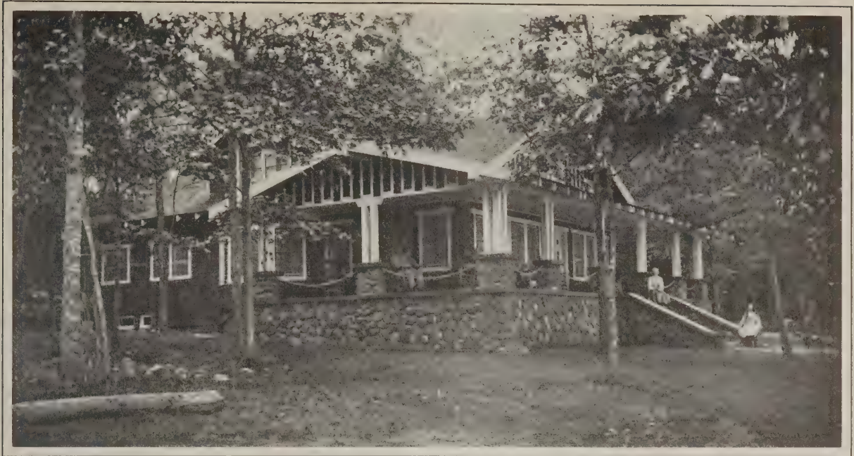
Summer Cottage in the Maine Woods of Mr. J. K. Robinson of New York City—View Looking Toward the Left-Hand Front Corner of the Building
