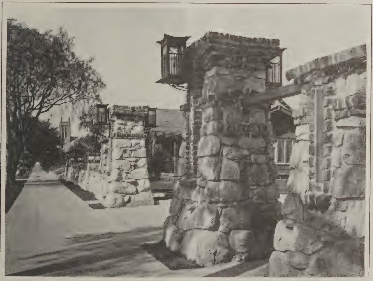
The Rustic Masonry of Local Stone, the Curious Belt Courses and the Quaint Lanterns at the Tops of the Gate Piers Give an Entrance That Is at Once Unique and Impressive
