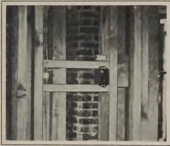
Residence Construction in Indiana—Fig. 11—Framing for Electric Wall Plug
