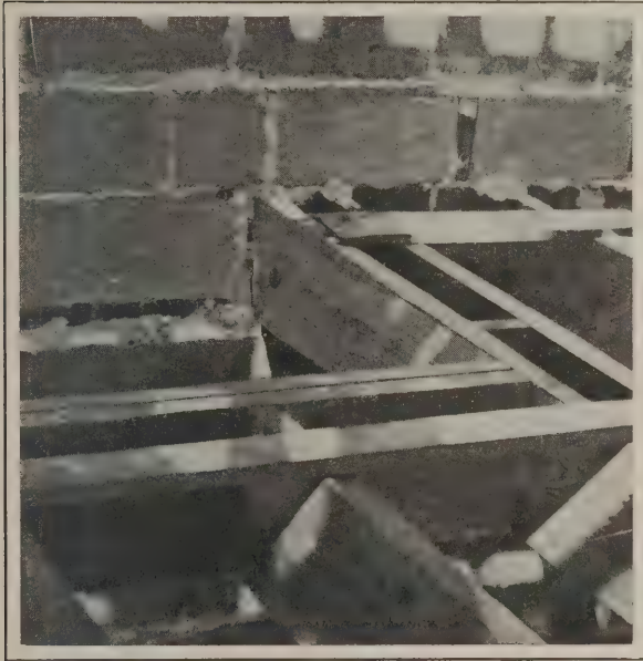
Fig. 4—View of Central Wall and Floor Joist
