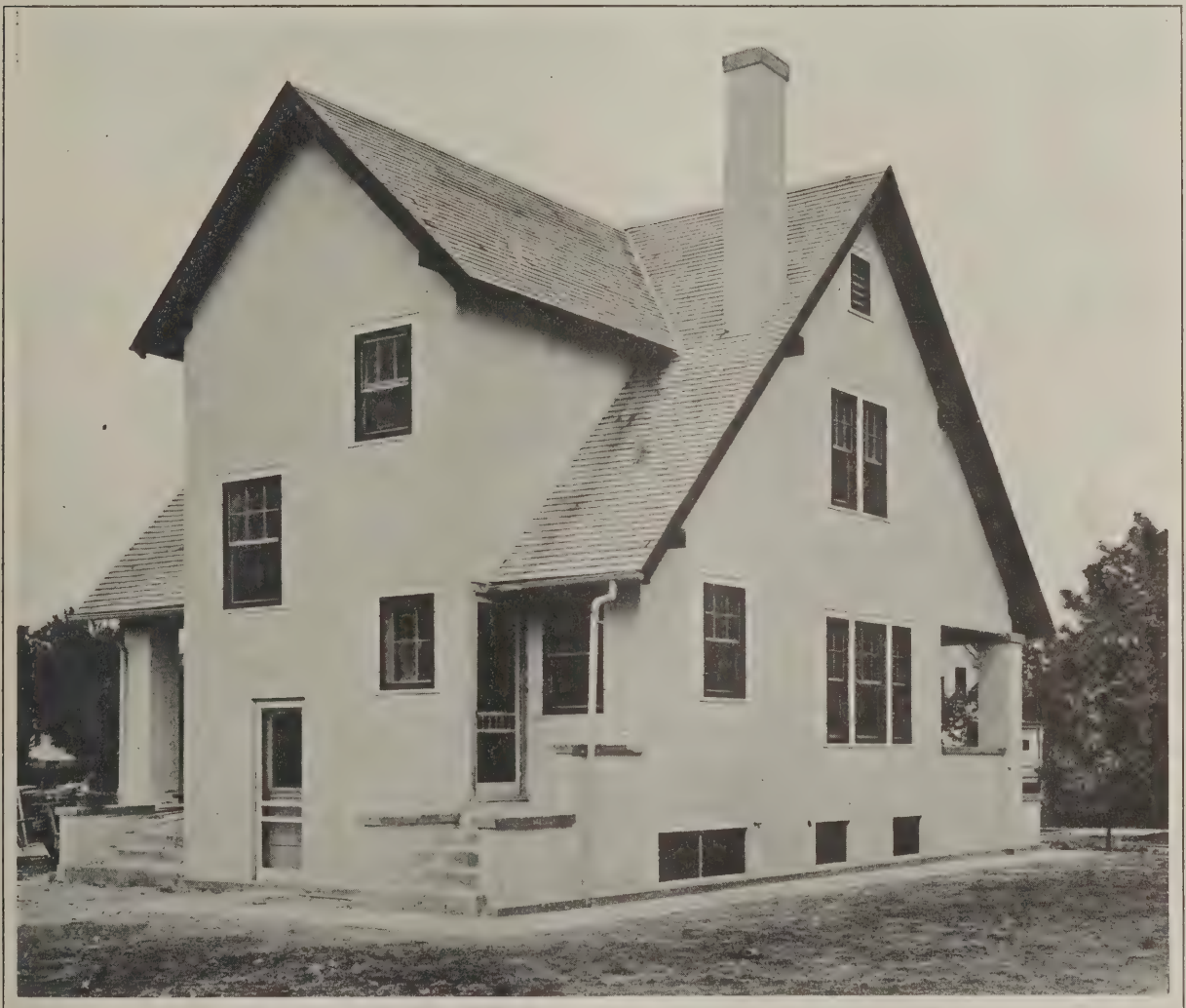
A Suburban Home of Tile and Stucco—The Rear and Side Elevations Showing Grade Entrance As Well As Porch Entrances to Kitchen and Living Room
