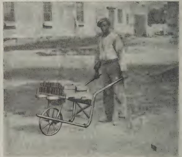
Fig. 3—Carrying Brick to the Job
