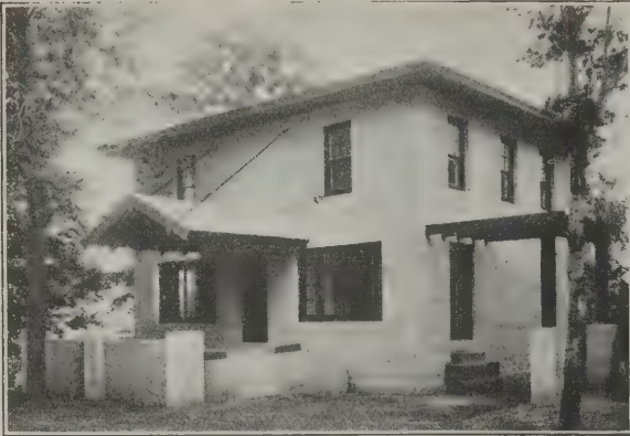
Erected with Van Guilder Hollow Wall Concrete Machine
