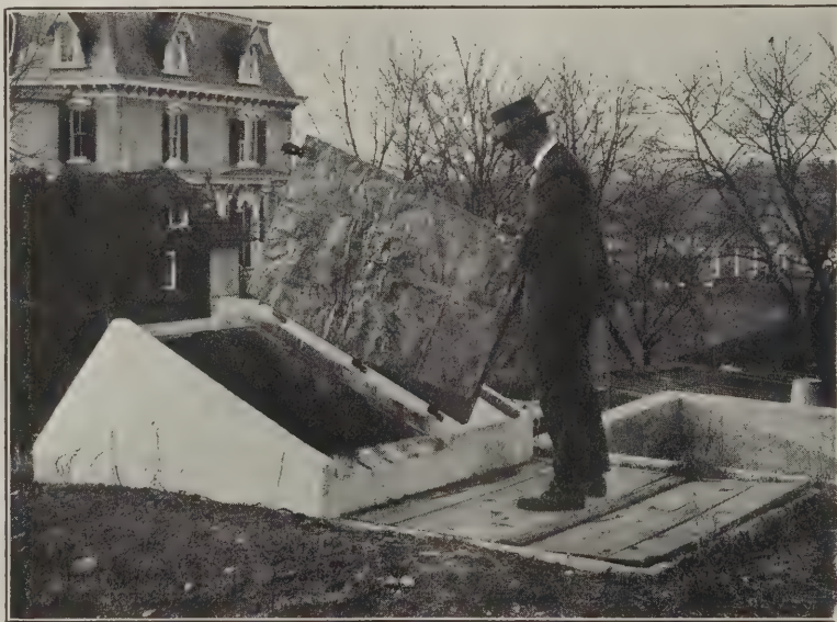
A Concrete Cellar for an Acetylene-Generator at Chalfonte, Pa.
