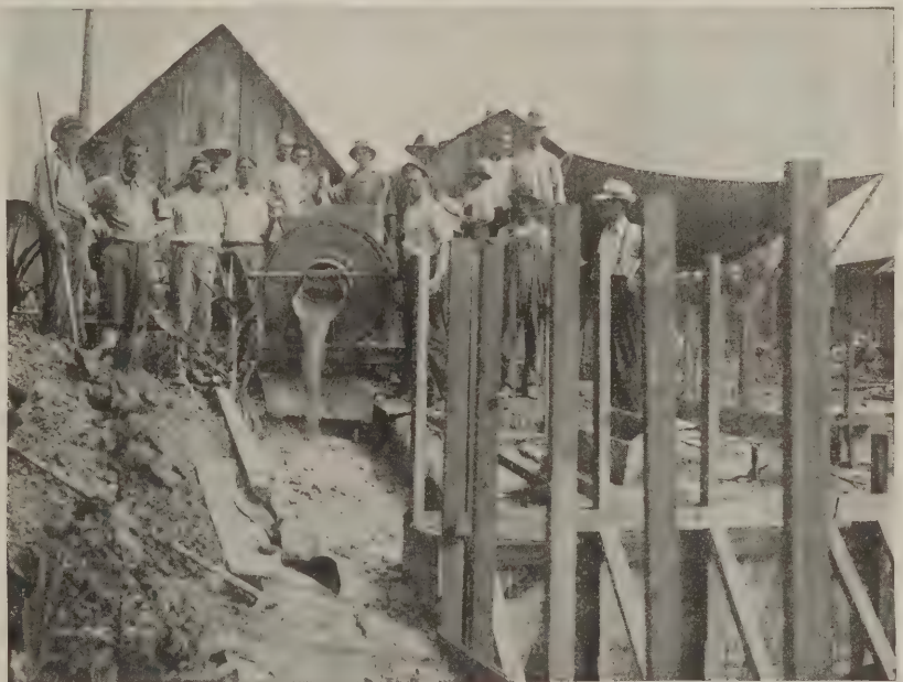
“Little Devil” Mixer on Two Wheels, with Charging Spout.
