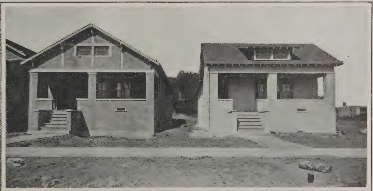
TWO DIFFERENT TYPES OF TILE HOUSES AS THEY APPEAR WITH THE STUCCO APPLIED TO THE EXTERIOR SURFACES
