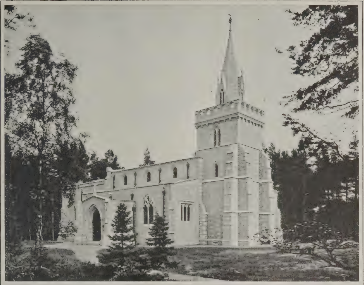
Exterior View of Aboyne Church Showing Broken Squared Dressed Rubble Work
