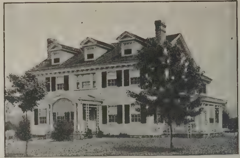
Walls finished with Cabot's Old Virginia White Roof finished with Cabot's Creosote Stain
