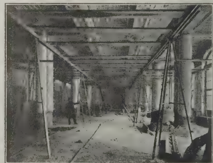
Fig. 8—The Scaffolding in Practical Use
