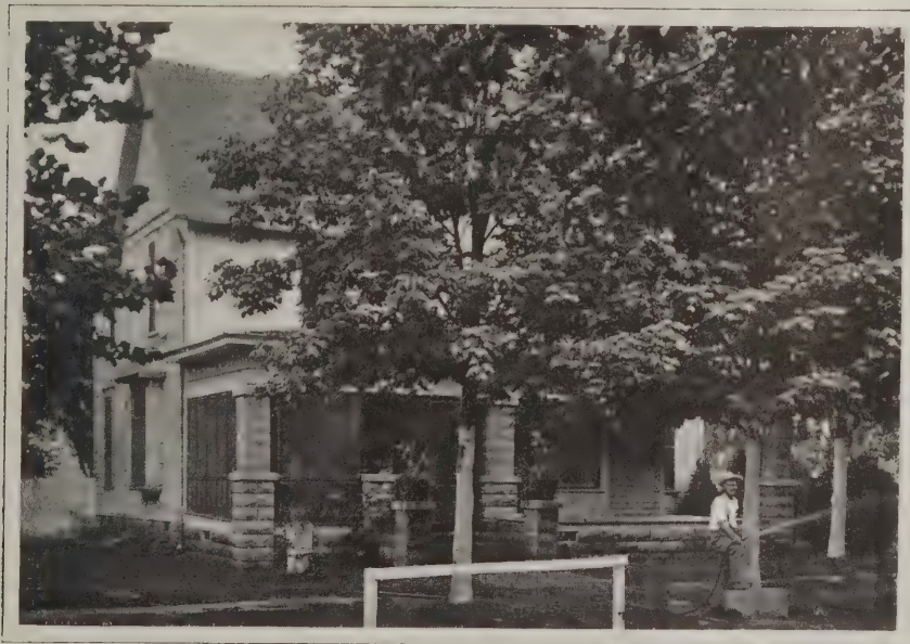
General View of the House With the Owner Shown Sprinkling the Lawn
