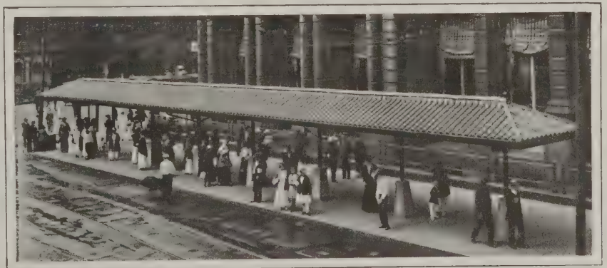
Fig. 2—Trolley Station Covered with Edwards Sheet Metal Tile
