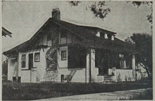
The Cottage of a Chicago Builder from November Building Age. W. K. Johnston, Architect, Chicago: "... before laying the shingles were dipped in Cabot's Green Creosote Stain."
