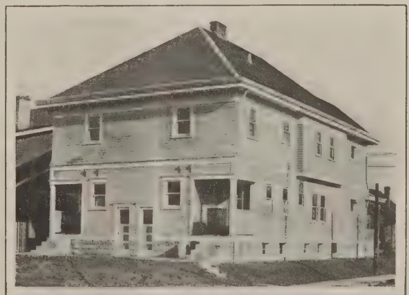
Fig. 12—Rear View of the Completed House
