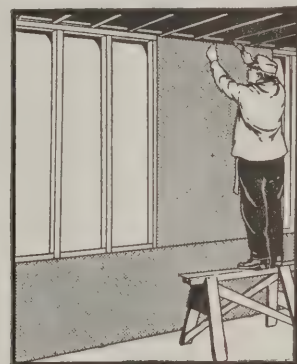
Start at top and nail to intermediate studding, before nailing edges. Use fine wire brads.
