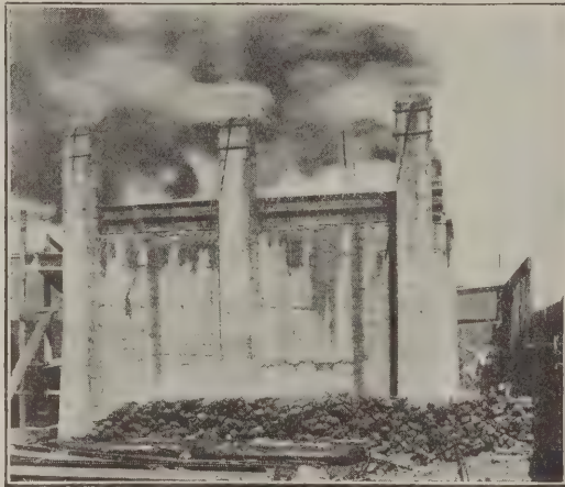
Test house during the fire. Note presence of excessive moisture
