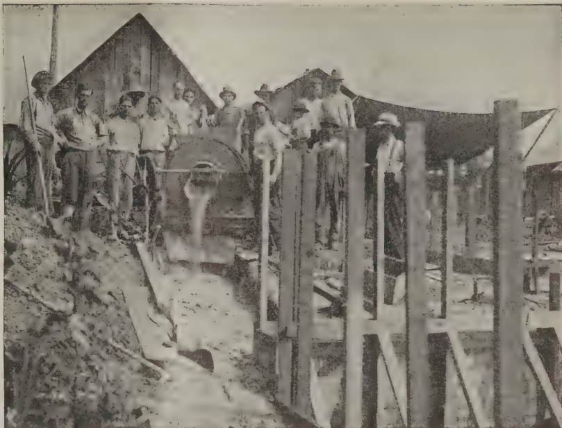
"Little Devil" Mixer on Two Wheels, with Charging Spout.
