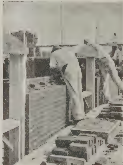
Figs. 7 and 8—Views Taken on the Scaffold Which Extends About the Building Showing the Way in Which the Materials Were Wheeled to the Various Benches Located at Intervals on the Scaffolding
