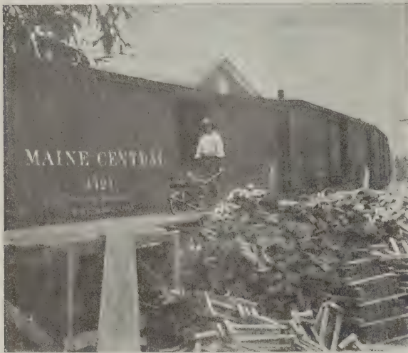
Fig. 1—Car Alongside the Brick Unloading Platform
