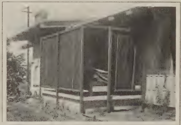
Fig. 3—Showing How Rolling Curtains May Be Used to Make the Sleeping Quarters More Private
