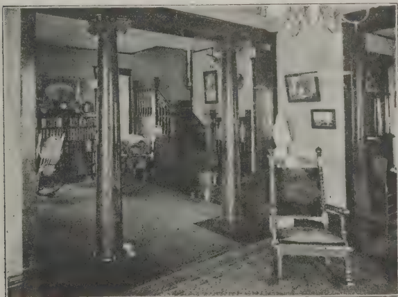
Fig. 2—Soft Pine as Used for Interior Trim, Stairs, Columns
