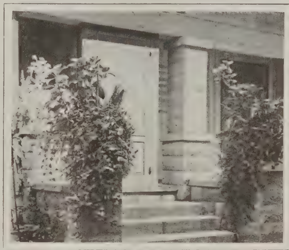
A Detail of the Front Entrance Showing the Concrete Block Foundation and Column Work
