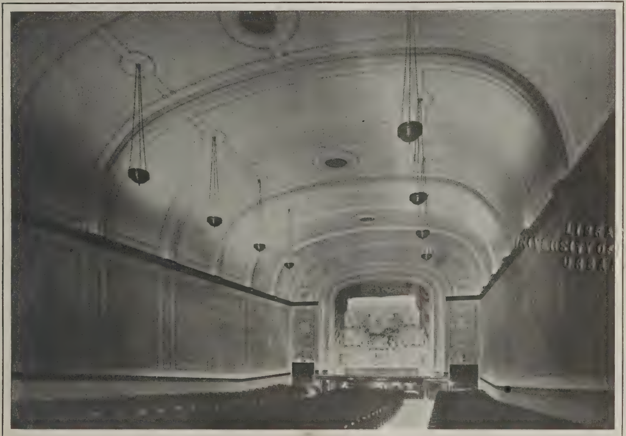
A Modern Moving Picture Theatre—Interior View Looking Toward the Stage and Showing the Two Exits at Right and Left of It; Also, the Two Intake-fan Openings Just Above the Cornice Each Side of the Proscenium Arch. Some of the Foul Air Vents are Seen in the Ceiling
