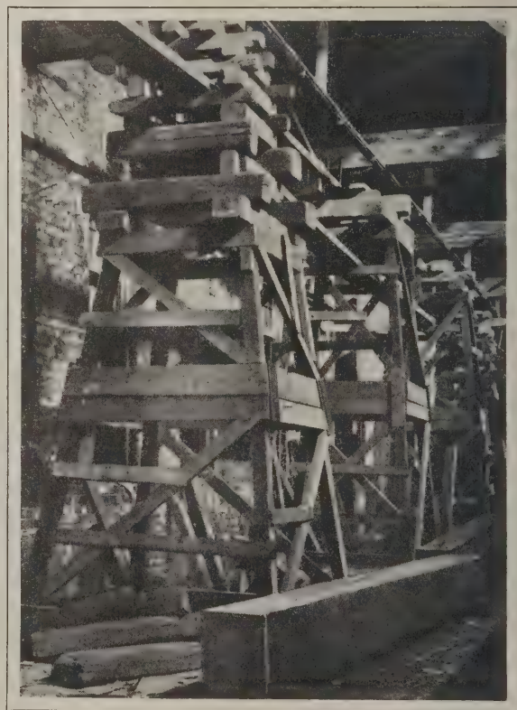
Fig. 6—Some of the Jack-Supporting Trestles
