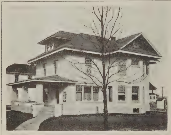
Van Gulden System of Hollow Wall Construction—Fig. 4—General View of Residence Built by this System
