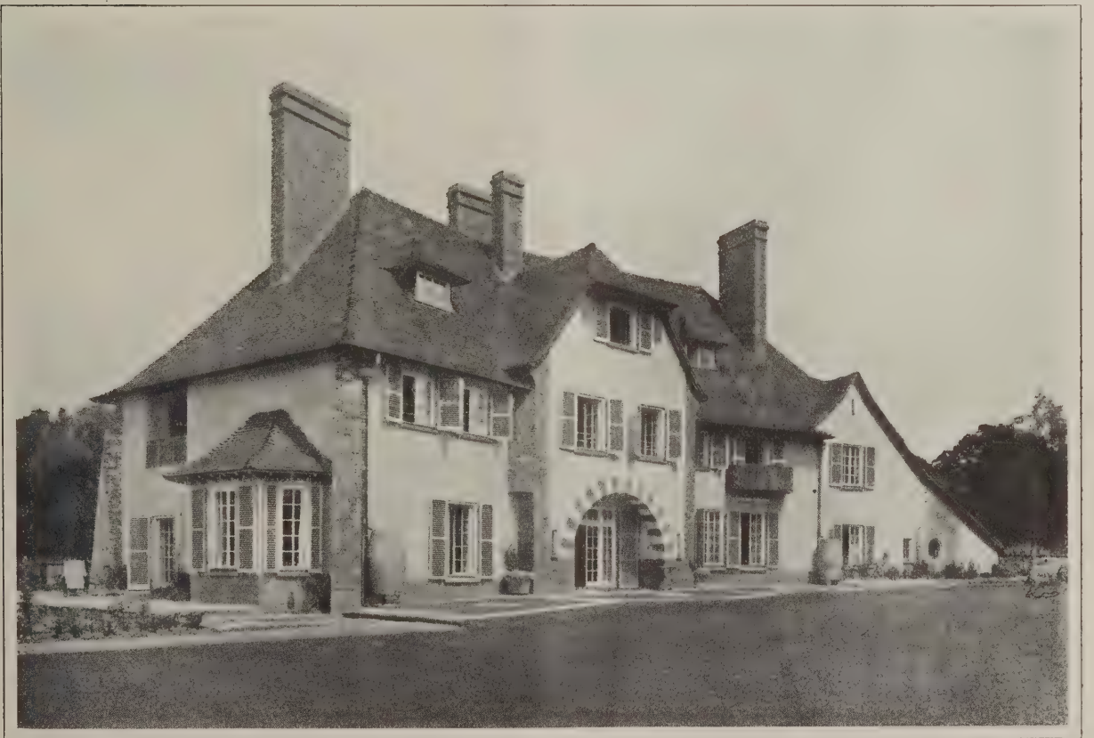
An English Summer Lodge Known as Pollards' Wood Grange, at Chalfont St. Giles, Buckinghamshire, England—The Entrance Front—Forbes & Tate, Architects
