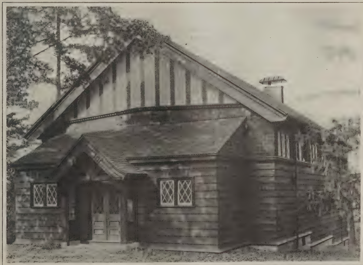
Gymnasium for an Industrial School at Fishkill-on-Hudson, N. Y.—Architects Allen & Collens, Boston, Mass.
