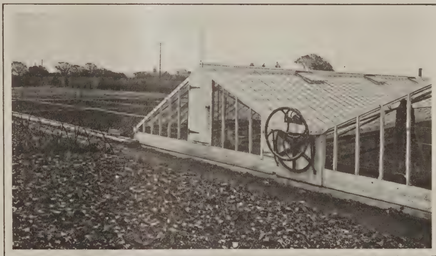
Construction of a Movable Greenhouse—Exterior View Showing Operating Gear
