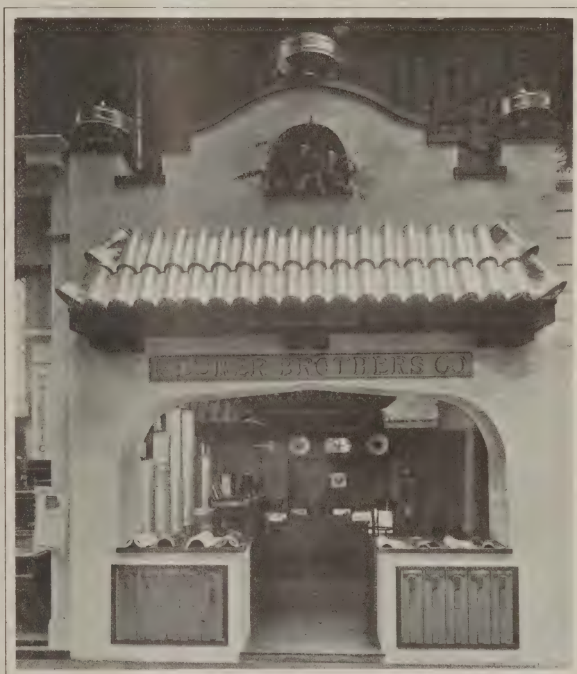
Fig. 1—A Sheet Metal Roofing Exhibit at the Panama-Pacific Exposition
