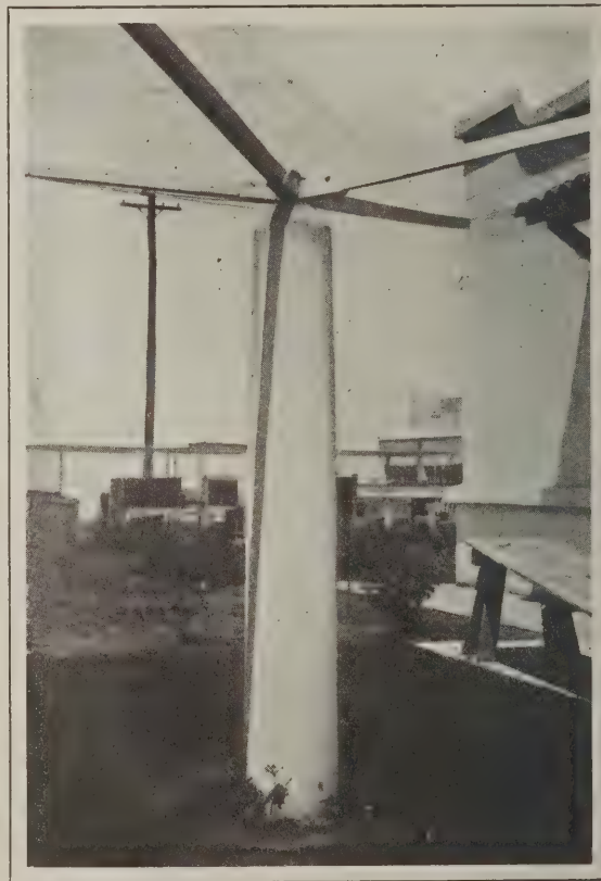
Cement Post for Clothes Dryer
