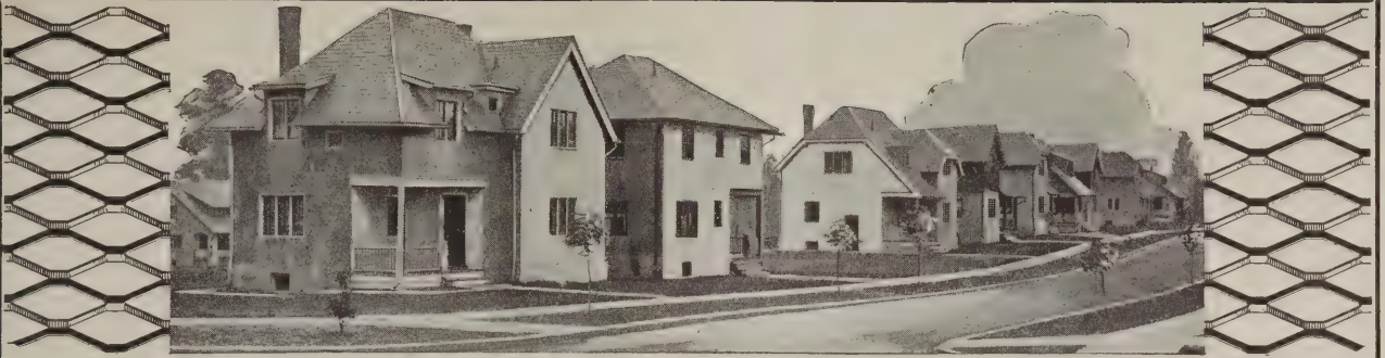
More than 100 Stucco Houses were erected in Akron, Ohio—Willis & Carley Co., Contractors. Sykes' Expanded Cup Self-Furring Metal Lath was used. Photo shows a few of these 100 houses.
