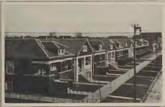
Fig. 1—Row of Houses Covered with International Asphalt Shingles
