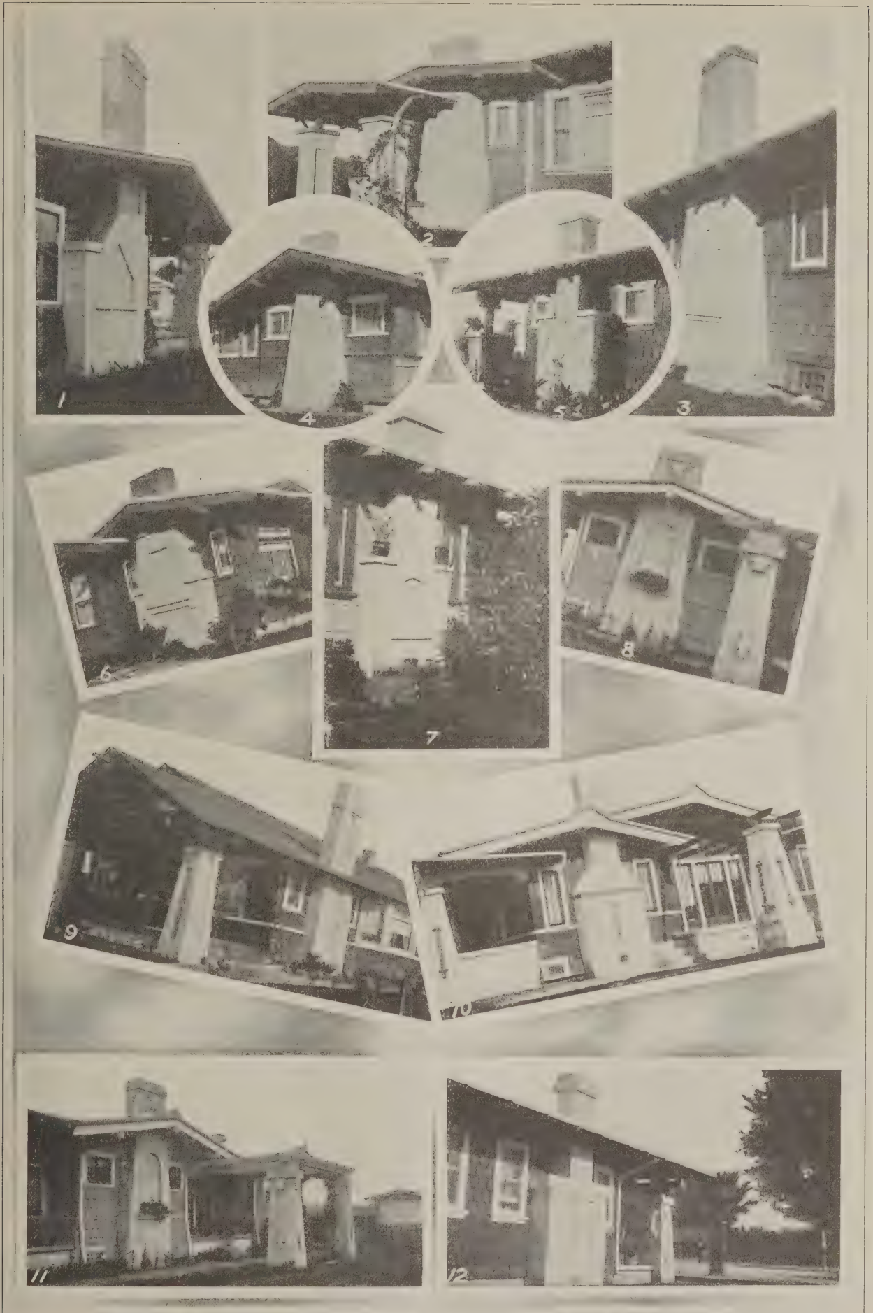
No. 1—Chimney with Sunken Panels; No. 2—Chimney for Low Buildings; No. 3—Tall Chimney of Semi-Plain Variety; No. 4—Chimney Whose Simplicity it Its Beauty; No. 5—Chimney Having Appearance of Cement-Block Construction; No. 6—Panelled Chimney with Flower Holders; No. 7—Block Chimney Showing Flower Holders Doing Service; No. 8—Side Views of Flower Holding Chimney; No. 9—Chimney with Stucco Finish and Deep Indentation; No. 10—Chimney Showing Effect of Brick Raised Work; No. 11—Near View of Flower Holding Chimney; No. 12—Another Block Chimney with Flower Holders.
