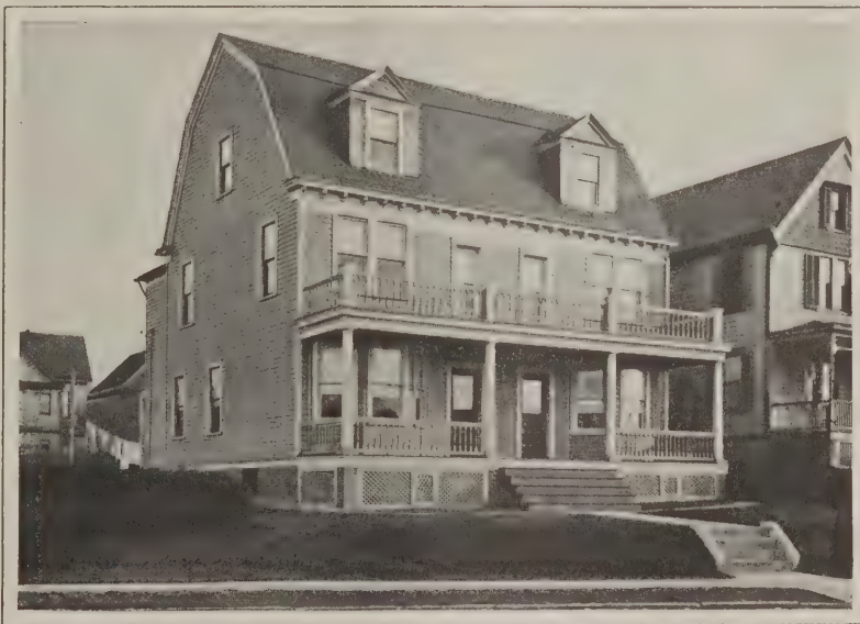
General Appearance of the Completed Structure
