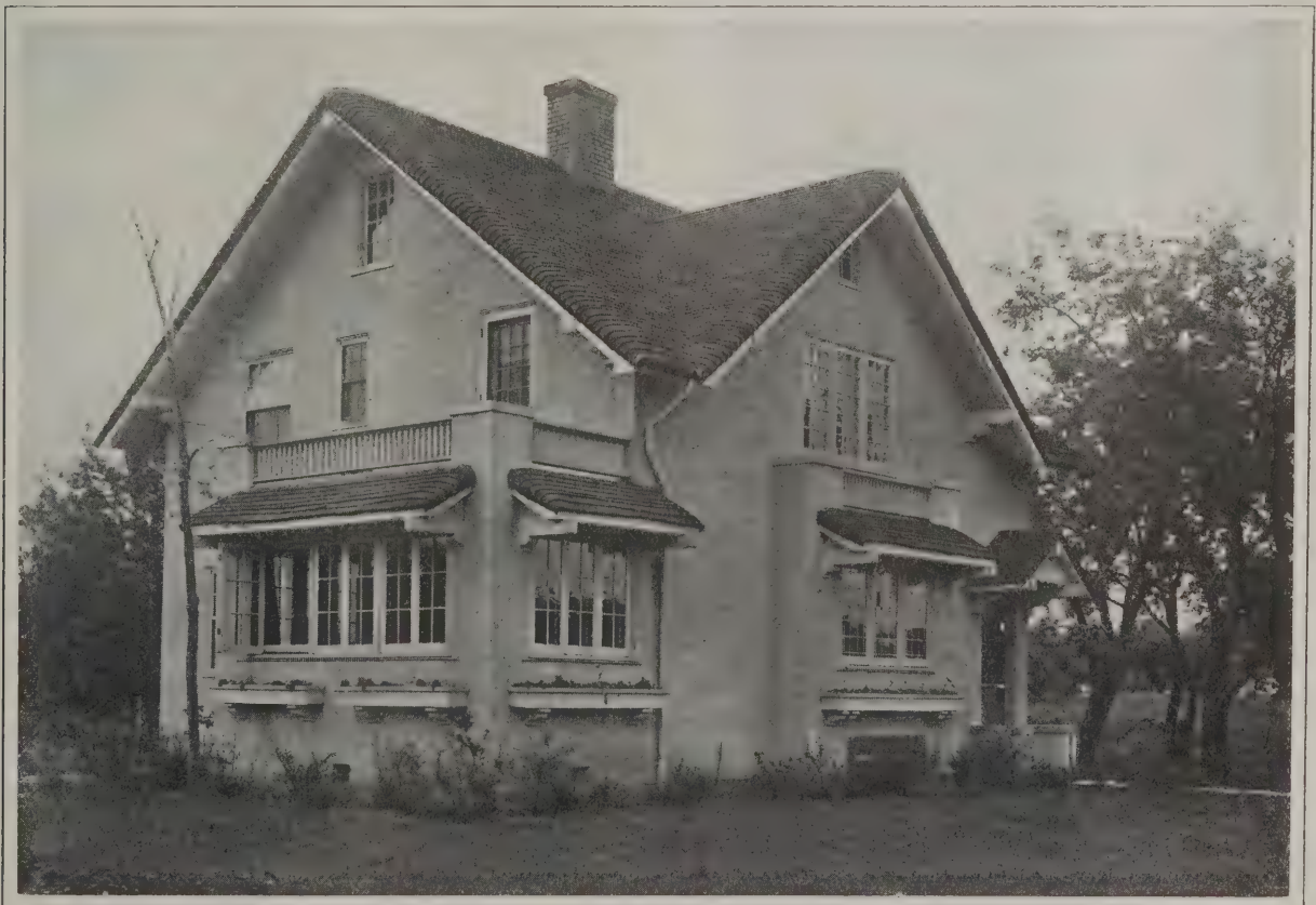
Another View of the Exterior of the House Showing the Sun Parlor; Also the Thatched Roof Effect
