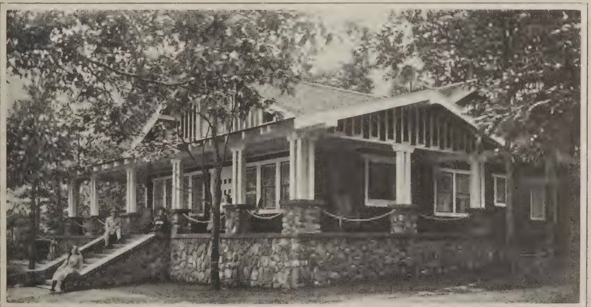
Another View of the Summer Cottage, Clearly Showing the Massive Stone Foundations
