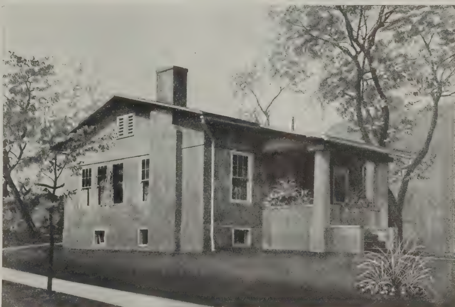
General View of One Side of Fireproof House Built of Cement and Steel
