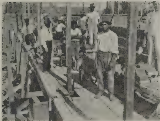
Figs. 7 and 8—Views Taken on the Scaffold Which Extends About the Building Showing the Way in Which the Materials Were Wheeled to the Various Benches Located at Intervals on the Scaffolding
