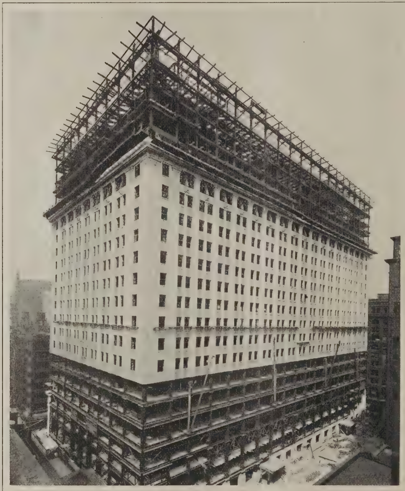
The Continental and Commercial Bank Building in Course of Erection
