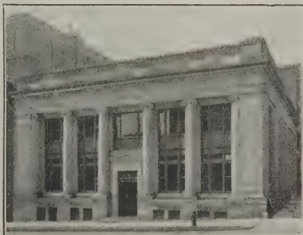
Detroit Fire and Marine Insurance Co. Roofed with Johns-Manville Built-Up Asbestos Roofing George E. Mason, Architect, Detroit
