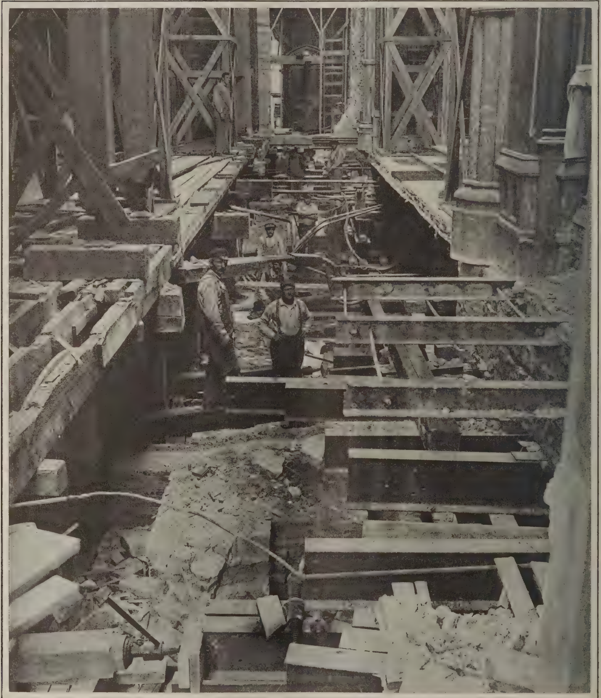
A Notable Church Remodeling Operation—Appearance of the Main Floor of the Building After the Rear Section Had Been Moved Back the Required Distance
