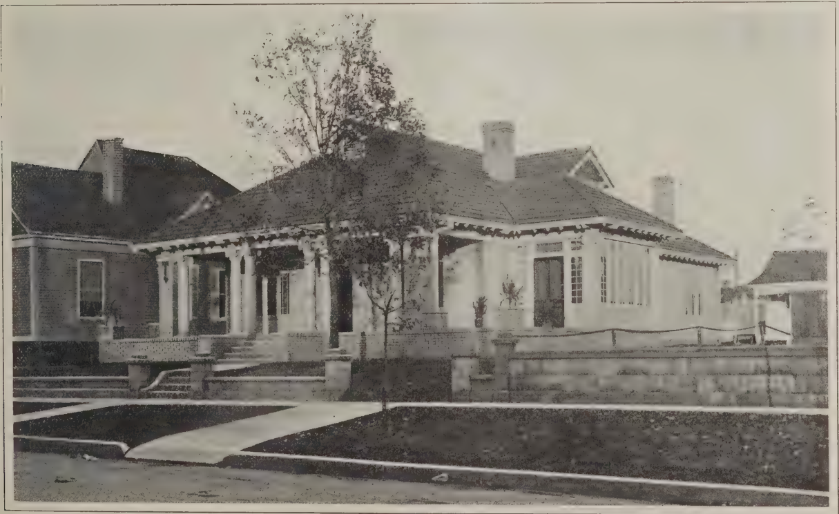
The Bungalow Residence of Isidore Lehman on South State Street, Jackson, Miss.—Architect, Emmett J. Hull of That City
