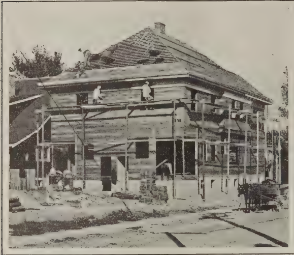
Fig. 8—The Painters Closely Following the Carpenters
