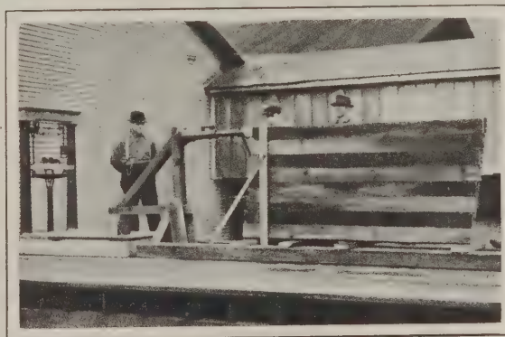
Fig. 3—Test of Section No. 2 Being Made
