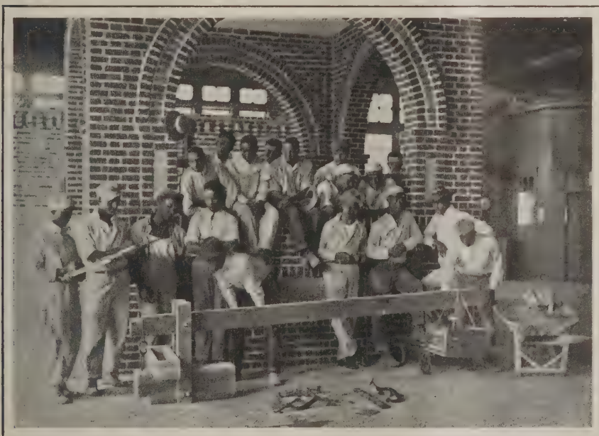
Fig. 1—Cement Testing at Hampton Institute with a Home-Made Machine
