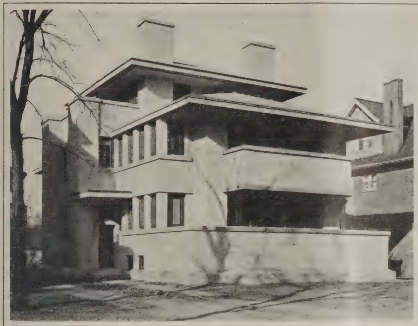
The Two-Family House of Hollow Tile—Front View of House Shown on the First Page of This Article
