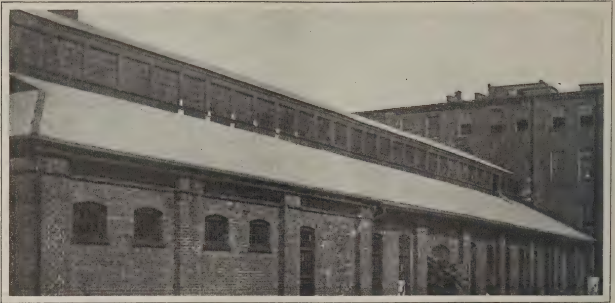
FIG. 1—GENERAL VIEW OF THE BUILDING BEFORE THE ROOF RAISING OPERATIONS HAD BEEN COMMENCED
