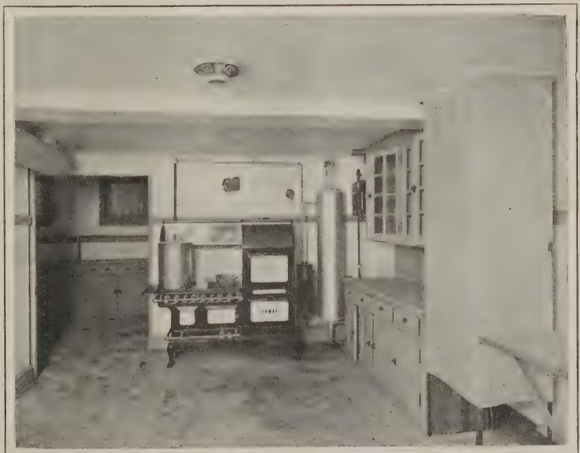
View in the Kitchen in Basement Showing Equipment and at the Right the Cold Air Duct from the First Floor
