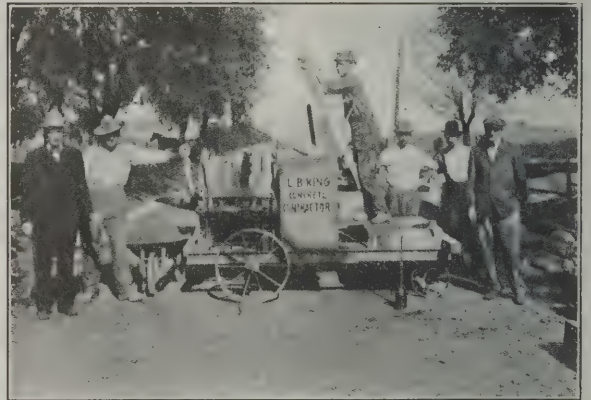
Fig. 6—The "Little Devil" Concrete Mixer in Use in Connection with the Building of Sidewalks
