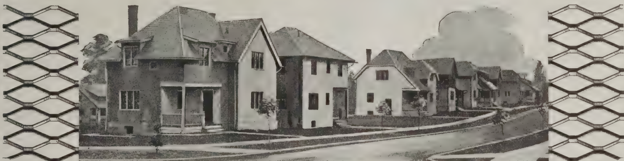
Stucco houses on Sprague Street, Akron, Ohio. A section of the Goodyear allotment on which Willis & Carley Company, Contractors, erected over 100 Stucco houses, using Sykes' Self-Furring Metal Lath.
