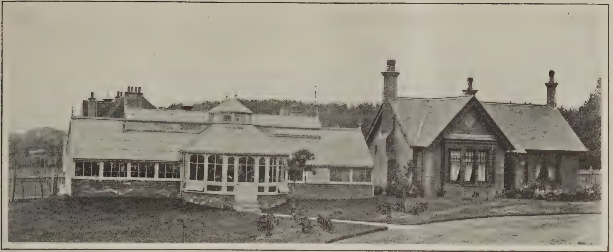
Features of the Modern Greenhouse—Fig. 2—A “Span” Greenhouse with Octagonal Bays in the Center of Each Side of the Structure
