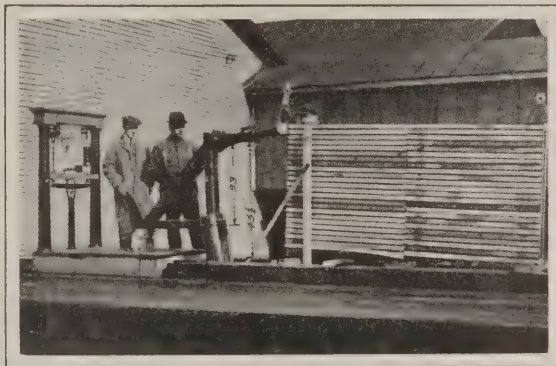
Fig. 2—Showing Test Section No. 1
