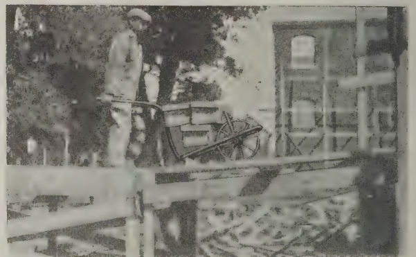
Fig. 4—Inclined Plane Leading to the Scaffolding Which Extends Around the Building
