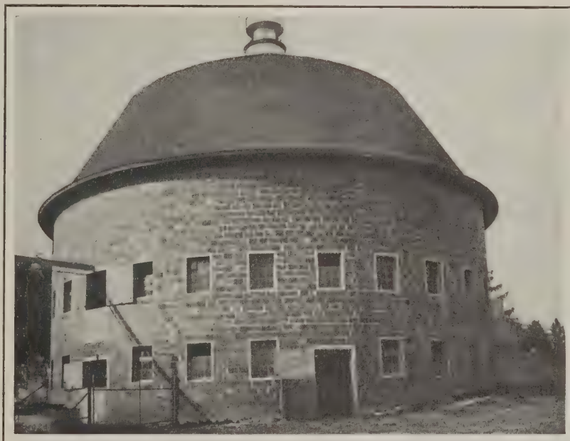
Appearance of the Barn as Viewed from the Point Indicated by the Arrow "A" on the Floor Plan on next page
