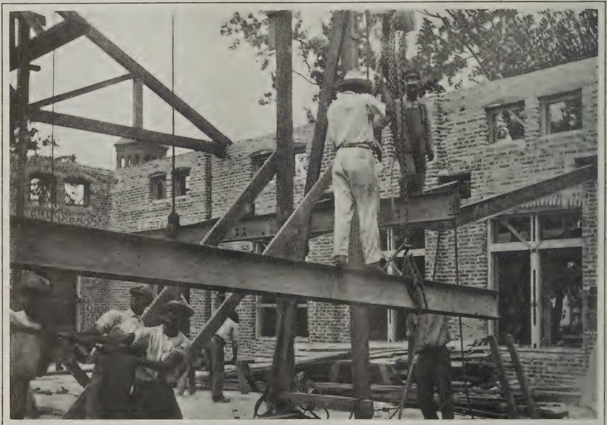
Industrial Education in the South—Fig. 7—Students at Hampton Institute Putting in Place the Iron Girders of Clarke Hall
