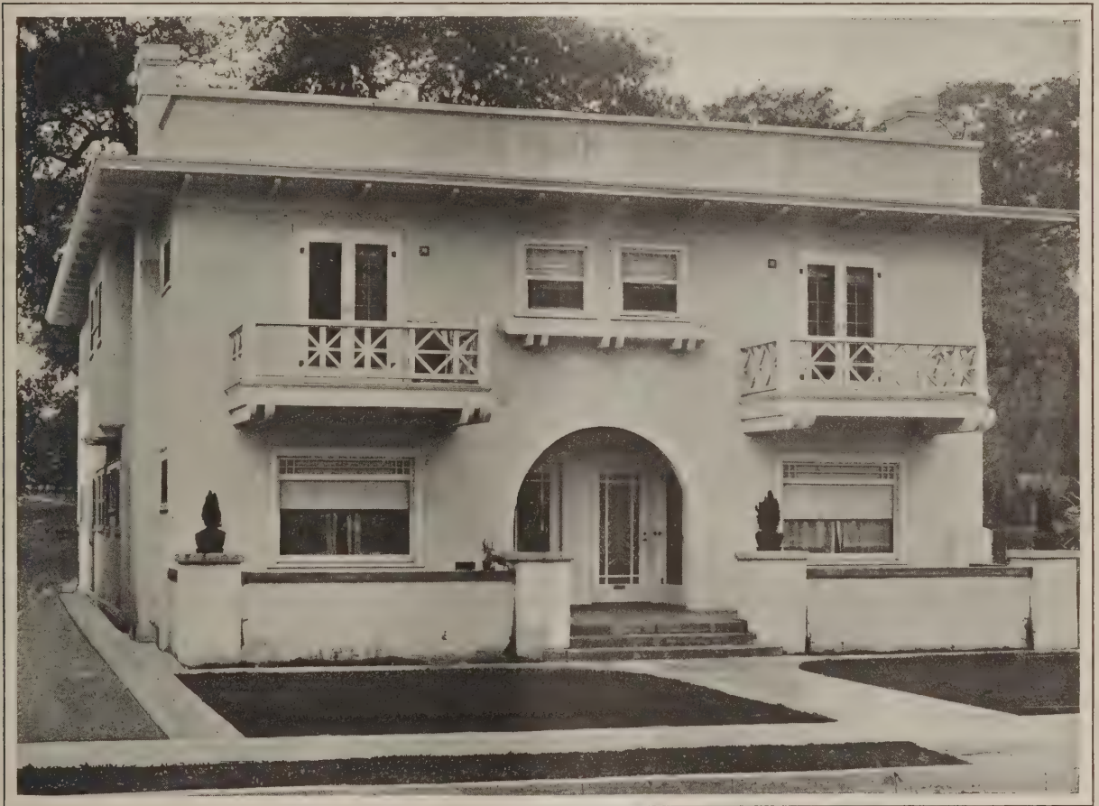
A Four-Family House of Stucco Finish—Architect, Rex D. Weston, Los Angeles, Cal.
