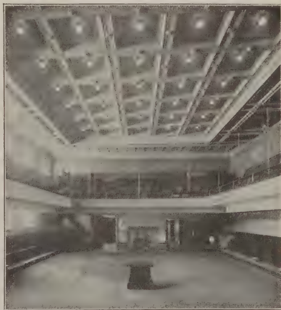
Fig. 2—Interior View of Lodge Room in Des Moines, Showing Berger's "Classik" Steel Ceiling
