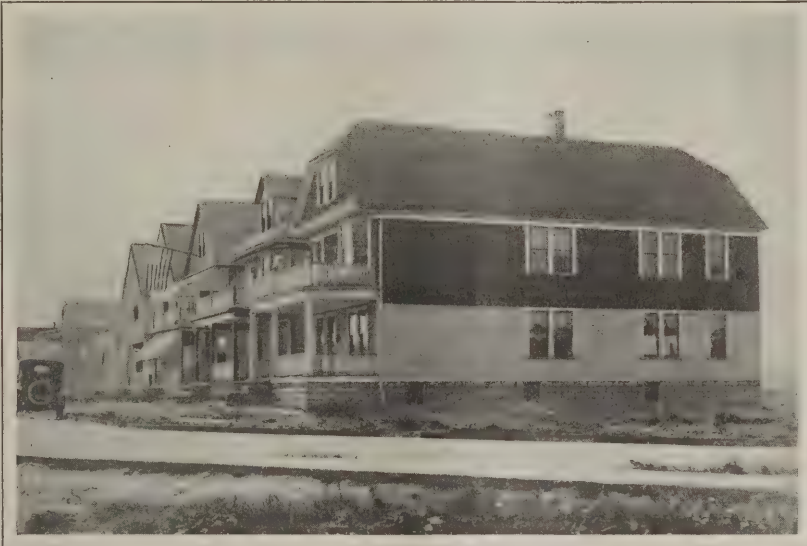
A Row of Two-Family Frame Houses with Floor Plans Below of the Building Shown in the Foreground
