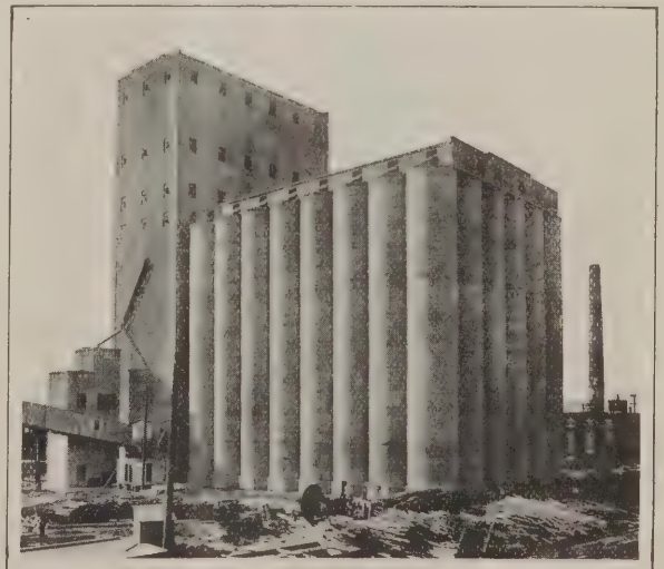
Fig. 2—Concrete Grain Elevator That Survived the Recent Galveston Cyclone
