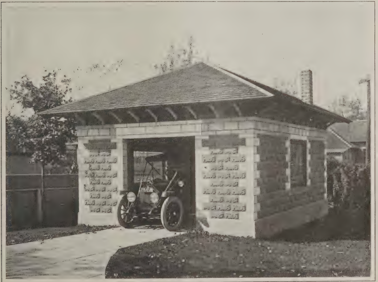
General View of a Garage Built of Concrete Blocks of Plain and Ornamental Face
