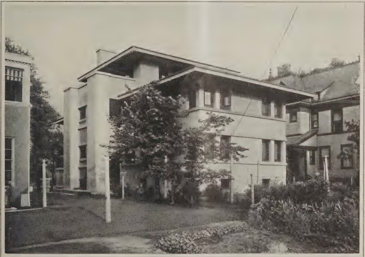
Two-Family Hollow Tile House of M. E. Bovee at Evanston, Ill.—The Garden Front Showing Immediate Surroundings—Architect, Walter Burley Griffin of Chicago, Ill.
