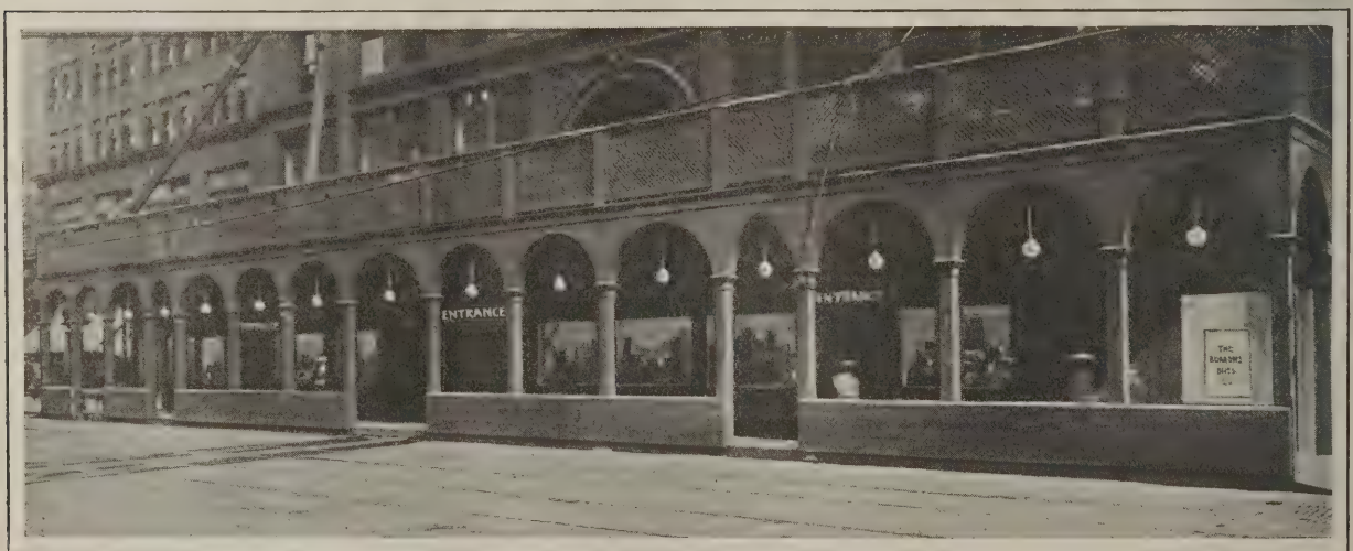
Sidewalk Shed in Front of a Cleveland Building During Alterations in the Façade
