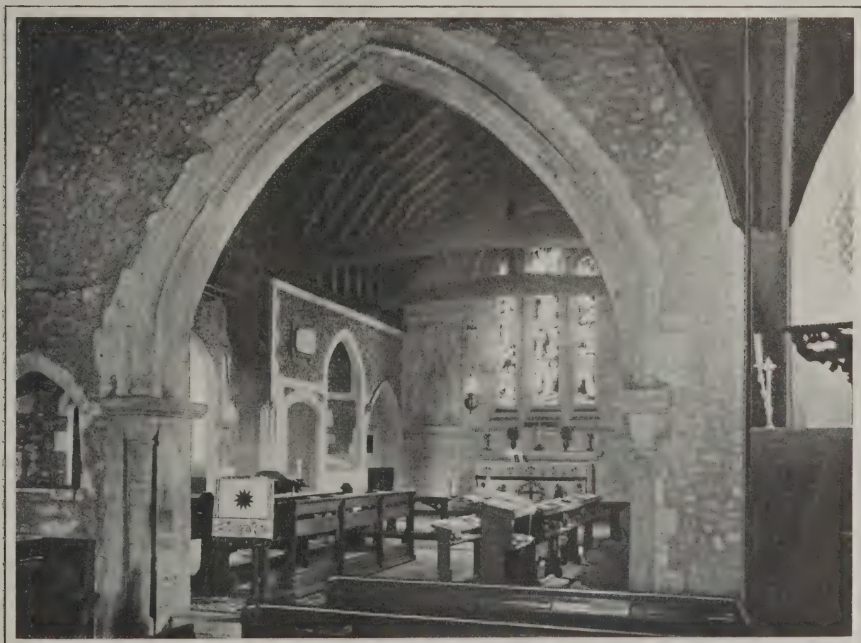
The Village Church in England—The Choir of Crawley Church with Trussed Roof and the Walls Built of Quartz Rock
