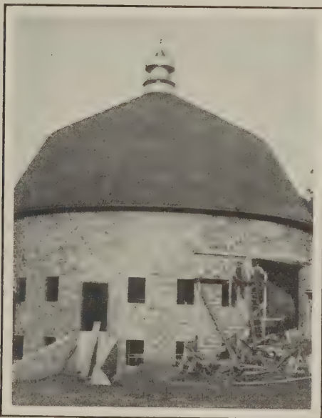
A Round Dairy Barn of Hollow Tile—Another View of the Structure
