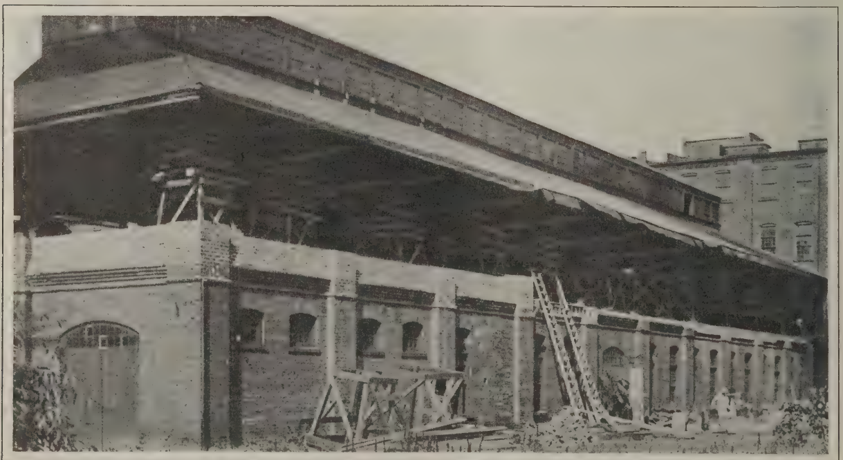
Fig. 2—Appearance of the Building After the Roof Had Been Raised to a Height of 13 Feet
