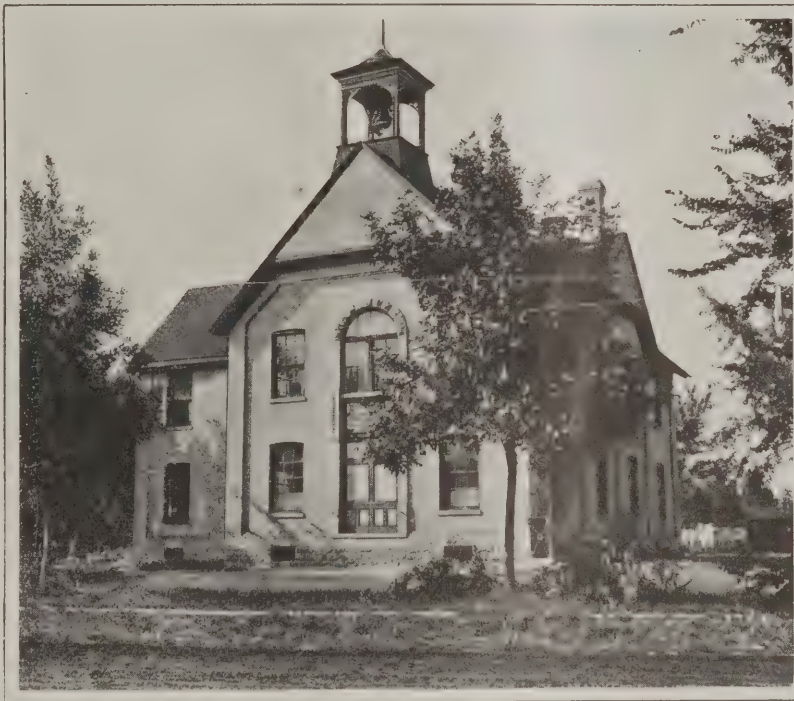
Heating a Two-Story Brick Schoolhouse—Fig. 1—General View of the Building and the Protection Afforded By Its Surroundings
