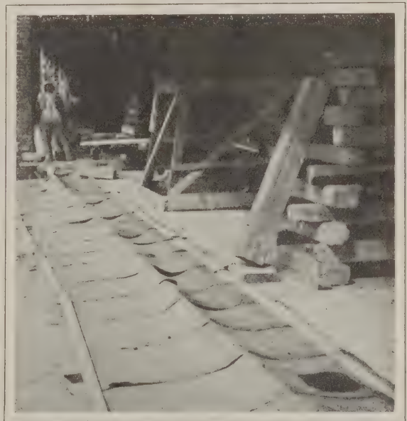
Fig. 8—Manner of Water-Proofing Over Contents of Building
