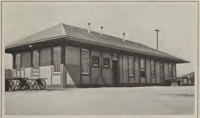
Fig. 6—The Appearance of the Railroad Station After It Had Been Completed
