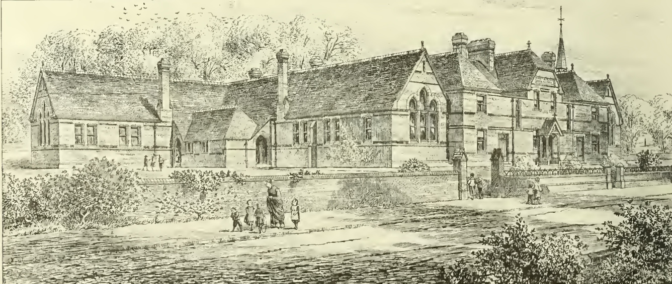
SCHOOLS AND RESIDENCE at BILLERICAY for the Great Burstead School Board. J. Edward K. Cullis Arch t
