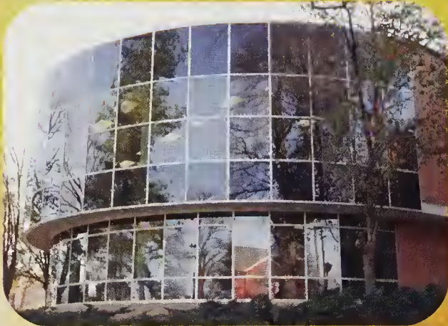
The outside of the café (which is on the second floor).
