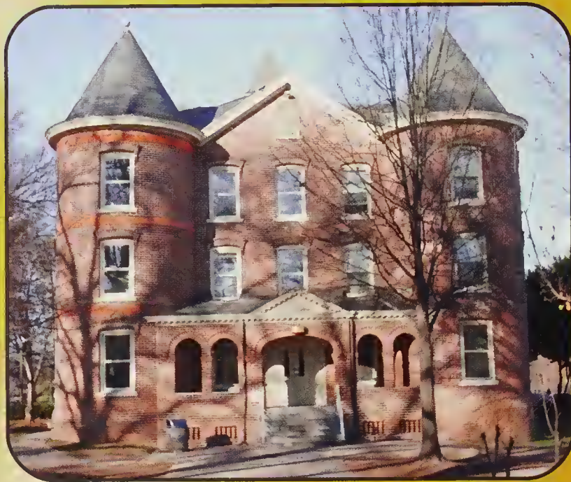
Carter Hall is the oldest residence hall on campus. It was constructed chiefly by students in 1896.
