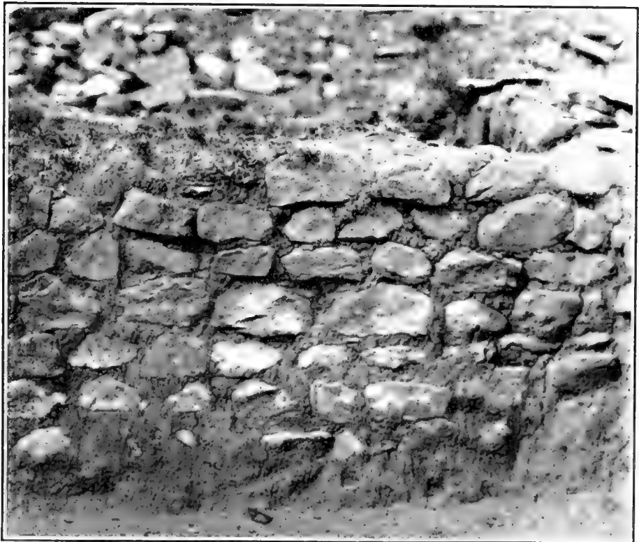
b. Characteristic stonework in later additions to house A
