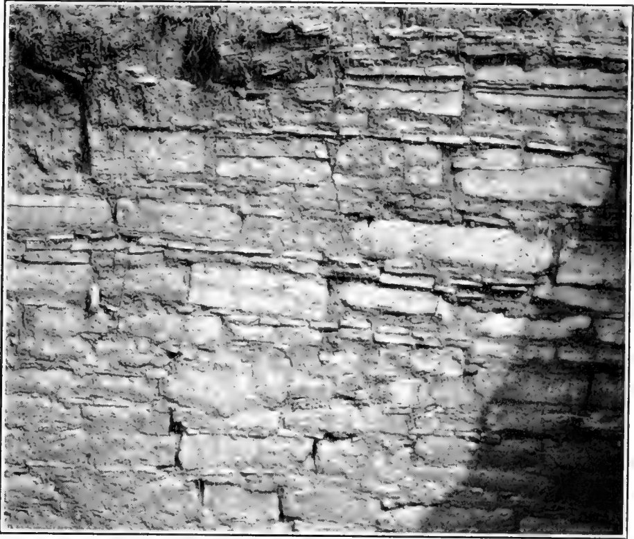
a. Wall construction in the old section of house A
