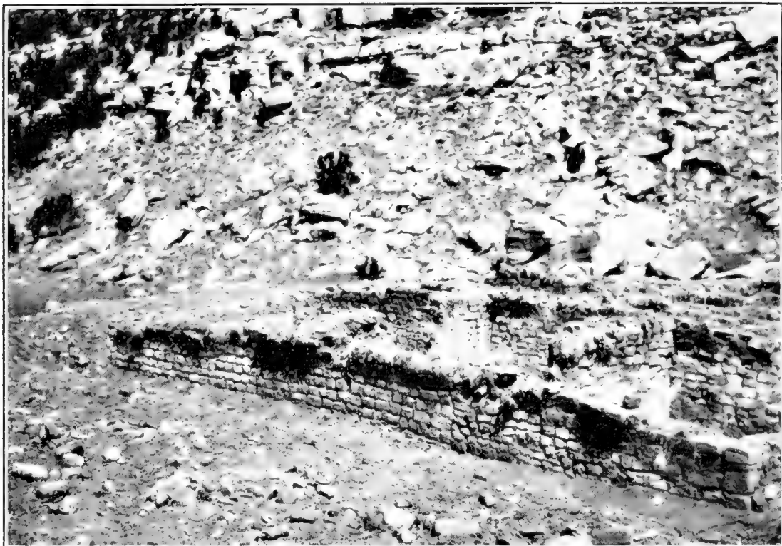
a. South end of building showing masonry
