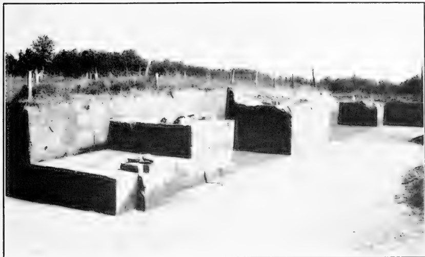
a , Method of excavating 30-foot profile, Site La° 13.
