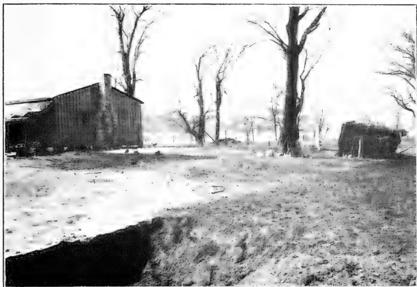
a, Excavation completed, trenches filled, Site Ma o 4.
