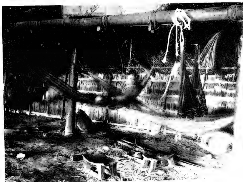
PLATE 93.—House types of the northwest Amazon. Top: Tucano house of the upper Papyon, Colombia. Bottom: Interior of a Baniva house. (Courtesy American Museum of Natural History.)
