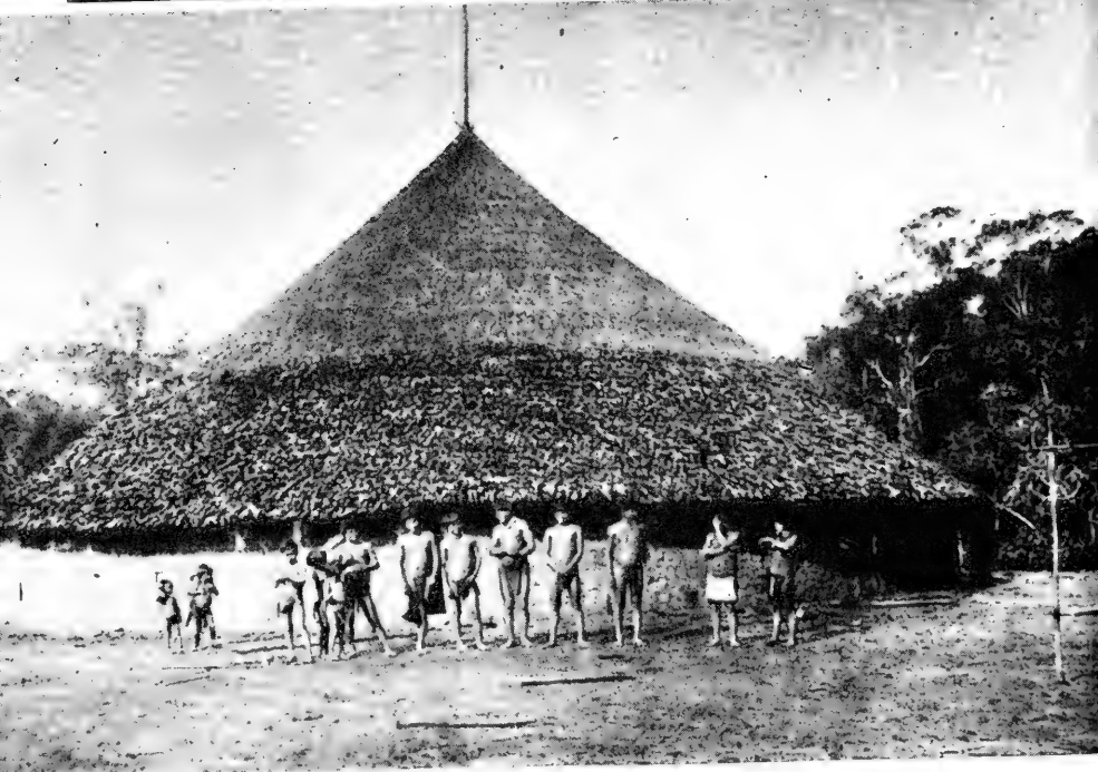
PLATE 108.—Guiana house construction. Top: Yecuana-Ihurana cone-shaped roof. The roof is covered from the inside out with palm leaves. Bottom: Completed hut. (After Koch-Grünberg, 1923 b.)
