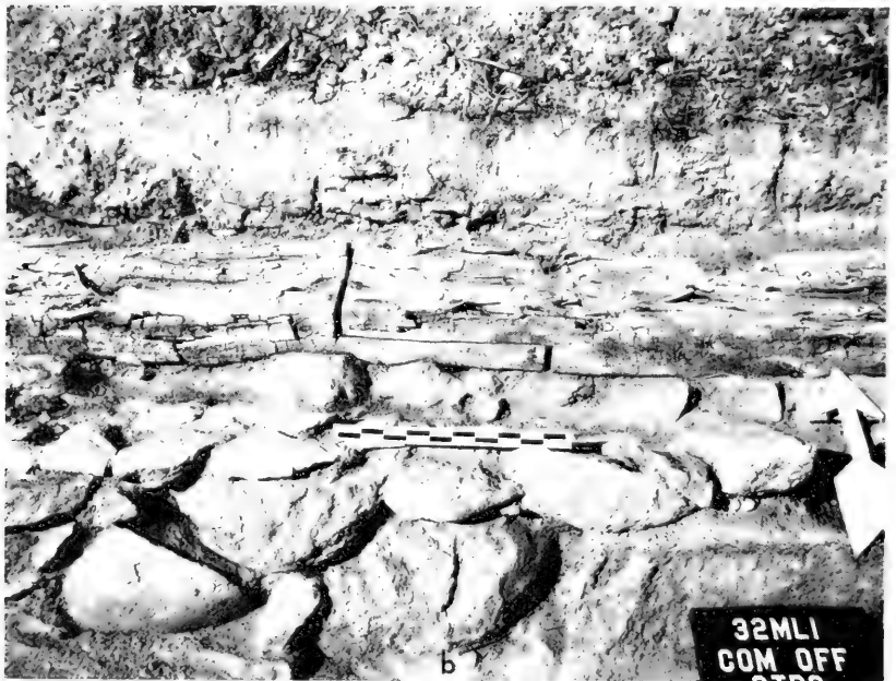
a , Detail of remnants of sills. Site of Commanding Officer's Quarters. b , Detail of lap joint in sills. Site of Commanding Officer's Quarters.
