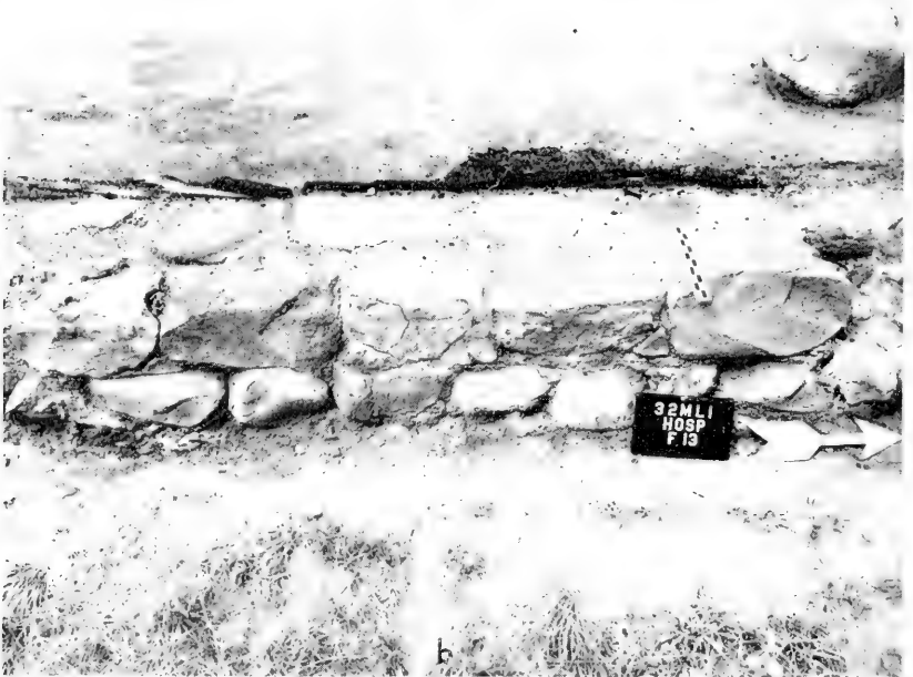
a , Interior view of footing of the northwest corner of the main body of the Hospital. b , Detail of stone masonry.
