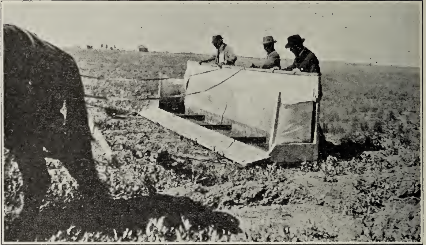
A hopper dozer in action. One of the many machines that was used in the grasshopper campaign, 1916, San Luis Valley. Note the hoppers in the pan. (Original).
