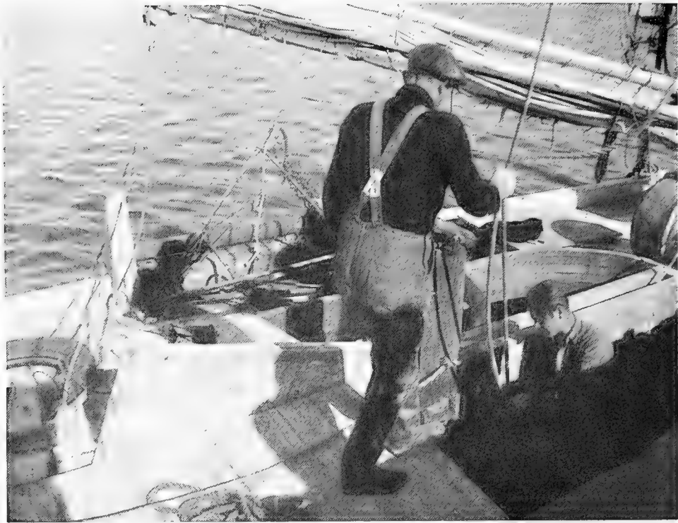
FIGURE 17.—Deck of a North Carolina sharpie schooner showing U-shaped main hatch typical of sharpies used in the Carolina Sounds.
