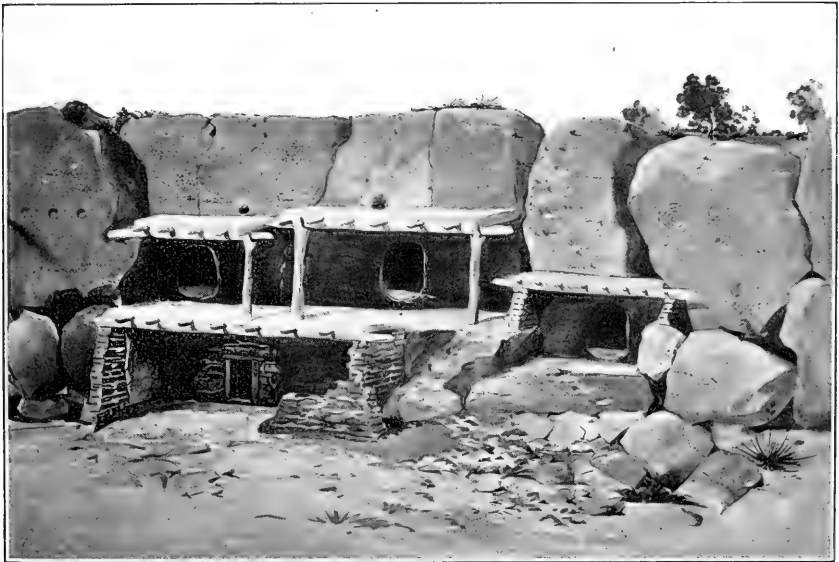
b RESTORATION OF CLIFF-DWELLINGS, TSHIREGE
