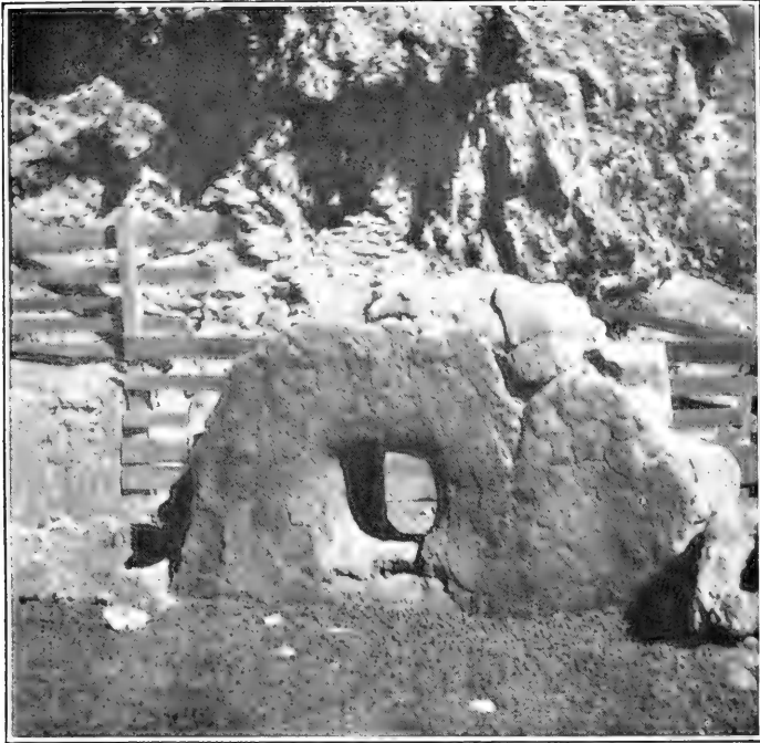
Remains of plastered walls
