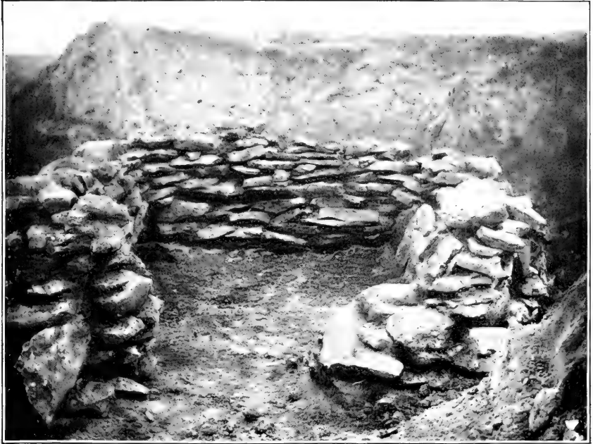
a LOOKING NORTHEAST THROUGH DOORWAY
