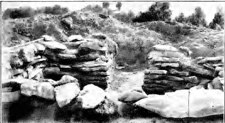
c DOORWAY IN VAULT
