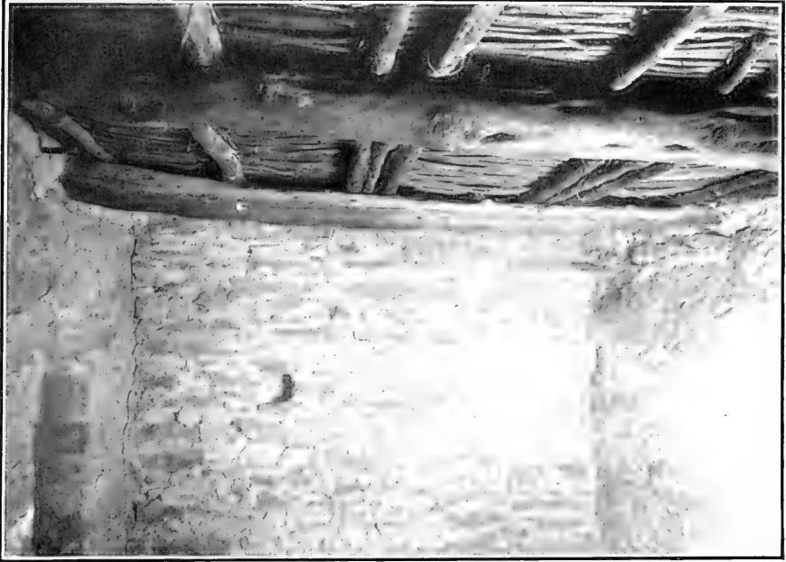
Roof of room 43
