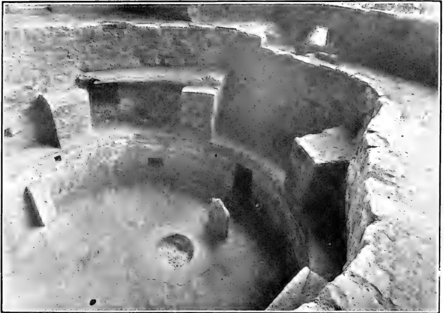
Kiva D, repaired
