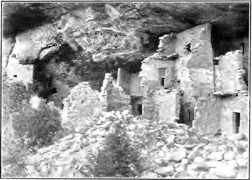
Plaza E. from the south, before repair
