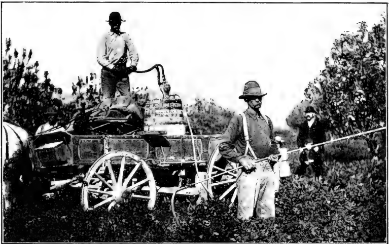
• FIG. 3.—HAND-POWER SPRAYING OUTFIT, IN WHICH THE PUMP IS MOUNTED UPON A BARREL ON AN ORDINARY WAGON.
