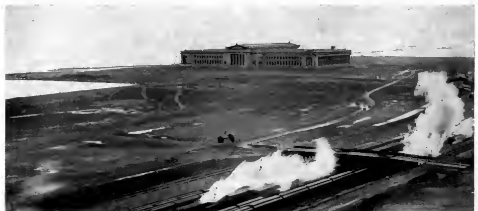
There were no other buildings. Shedd Aquarium, Soldier Field, and Adler Planetarium came much later.
