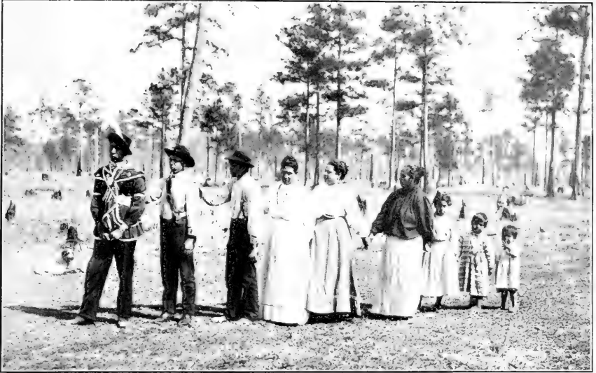
READY TO BEGIN
