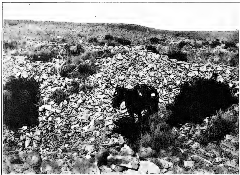
FIG. 89. Present appearance of the Wyoming quartzite quarries.
