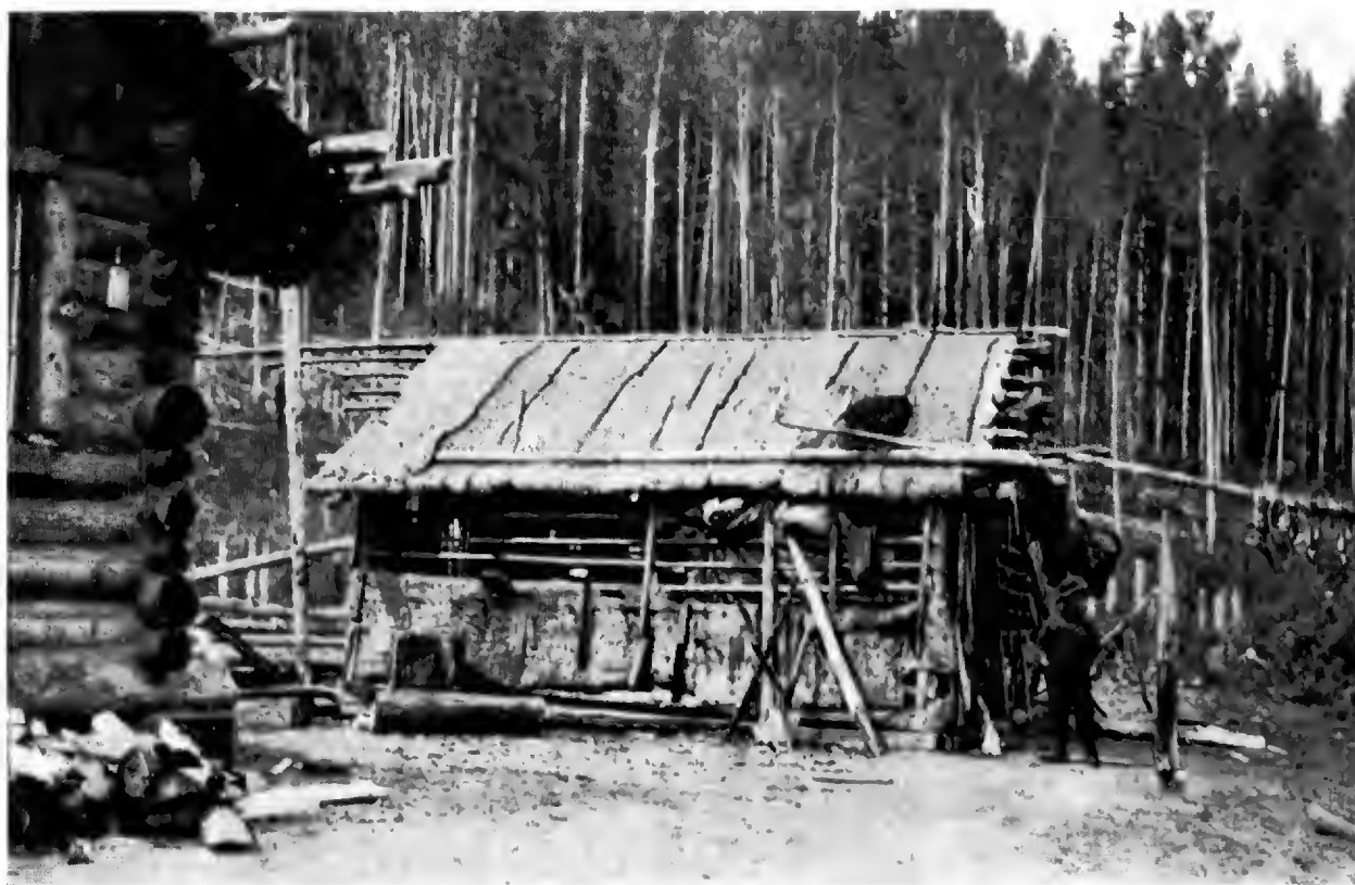
A Sekani hut of poles and spruce bark. ( Photo by D. Jenness. )
