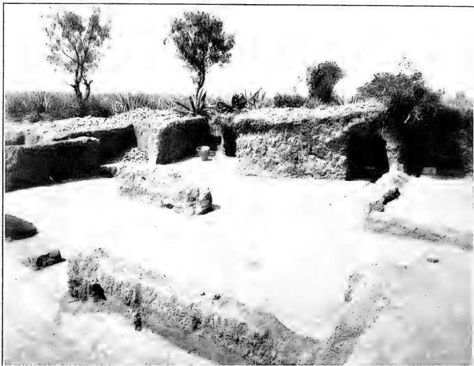
a. Southwestern corner of excavation, showing Room IX with foundations of pillars, Floor H, and Room X.
