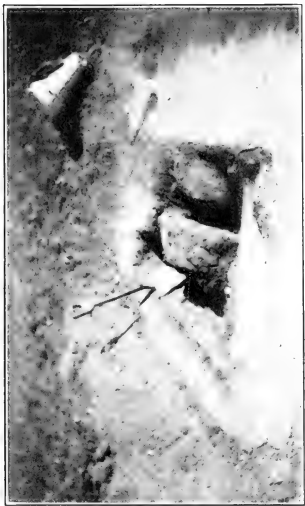
b. Floor A, break in floor, showing the upward slope at edges of floor.
