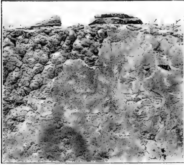
A. Wall construction, showing nodules.
