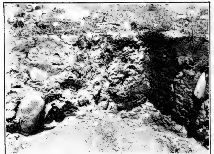
F. Cobblestone foundations.
