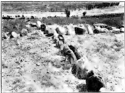
C. Foundation stones.
